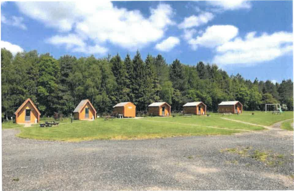
Fig.8 View from existing hardstanding area showing 5 glamping pods and facilities building, gravel pathways and grassy spaces. Note: proposed facilities building approximately in position of swing-set (right). Source: FWP
