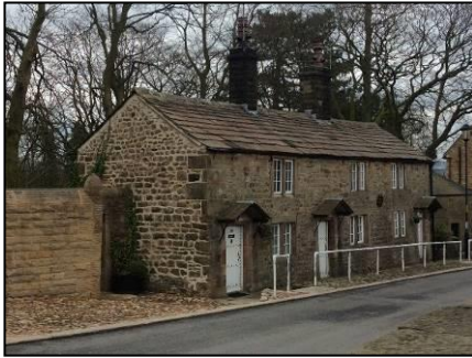
Fig.1: Elevations of farmhouse & lifted lead flashing prior to work
