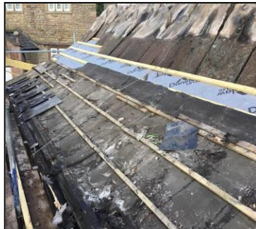
Fig.2: Initial stripping showed no evidence of roosting bats
