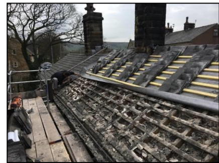
Fig.3: Loft void retained under newly laid felt
