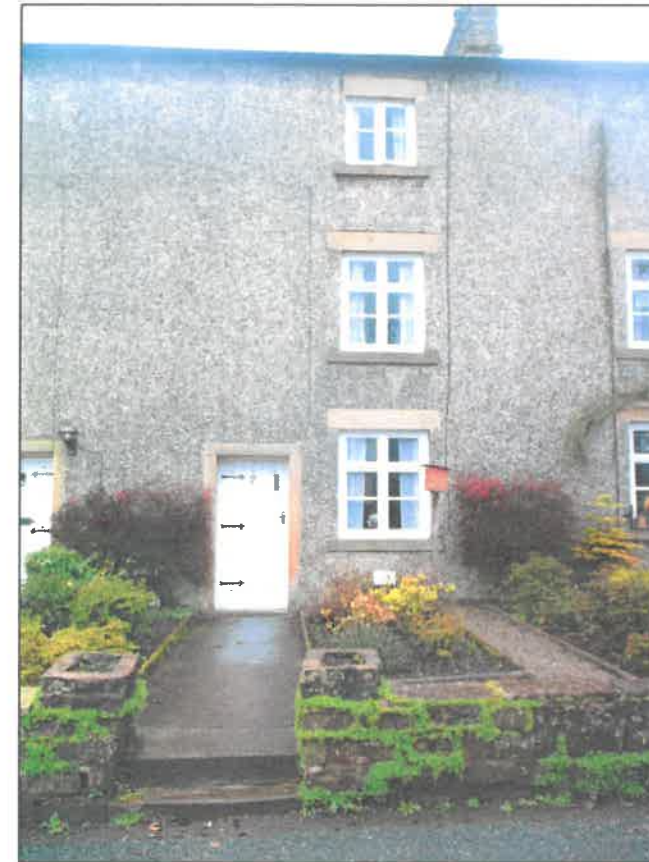
Left & Below: Slightly ramped concrete approach pathway to front door of house, steps up from the tarmac road surface.
