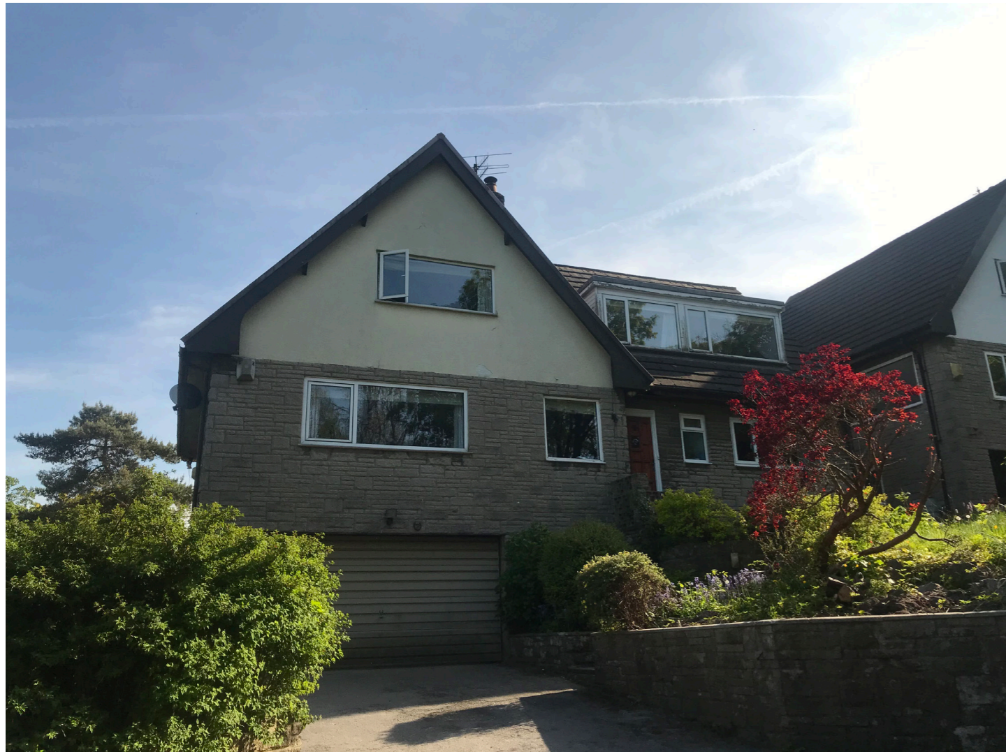
Existing principal elevation
