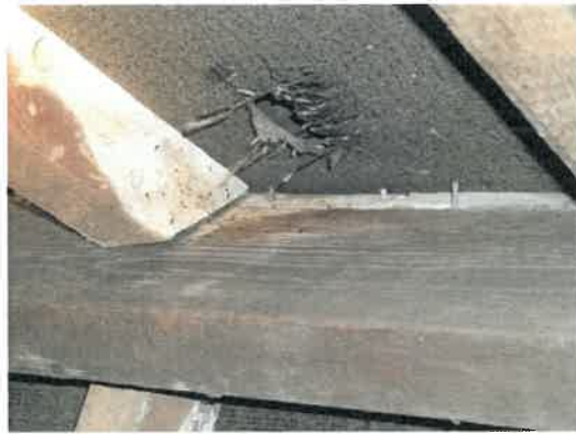
Plates 4 and 5. Bat droppings and tear in felt above, plus droppings on beam and rafter (zone 1)
