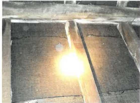
Plates 8 and 9. Bat droppings and over-lap in felt above (zone 5)
