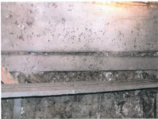
Plates 4 and 5. Bat droppings and tear in felt above, plus droppings on beam and rafter (zone 1)
