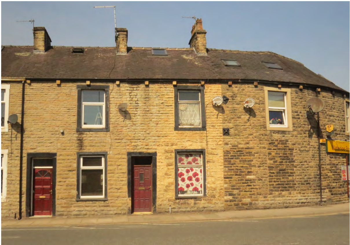
1 – The front of the house from Waterloo Road.
