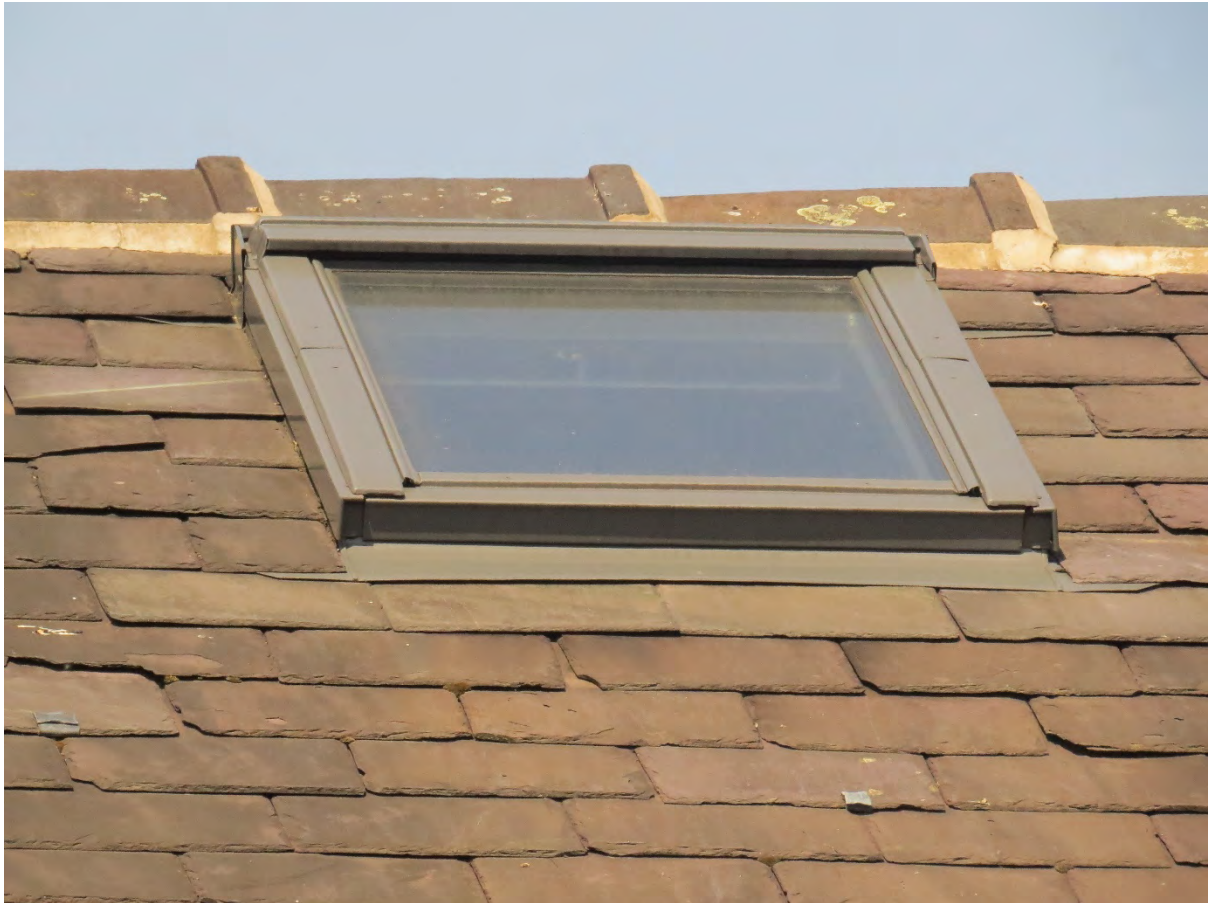
3 – The roof has a Velux roof light fitted.
