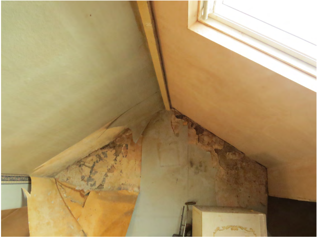
3.2a – The roof void.
