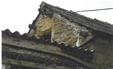
outbuilding gable and part shed roof
