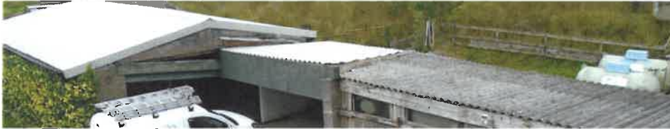
Garage and shed roofs
