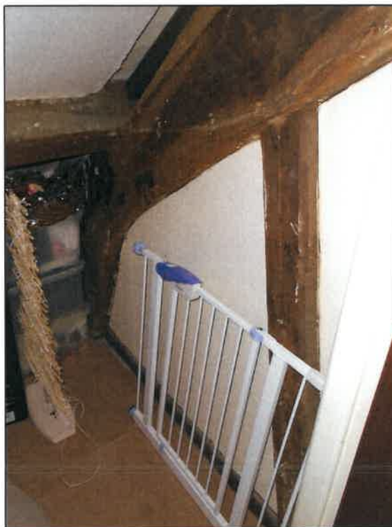
PL16: Upper cruck noted to the attic / second floor of the building
