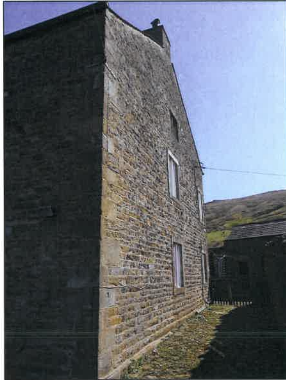
PL08: South facing elevation of the building
