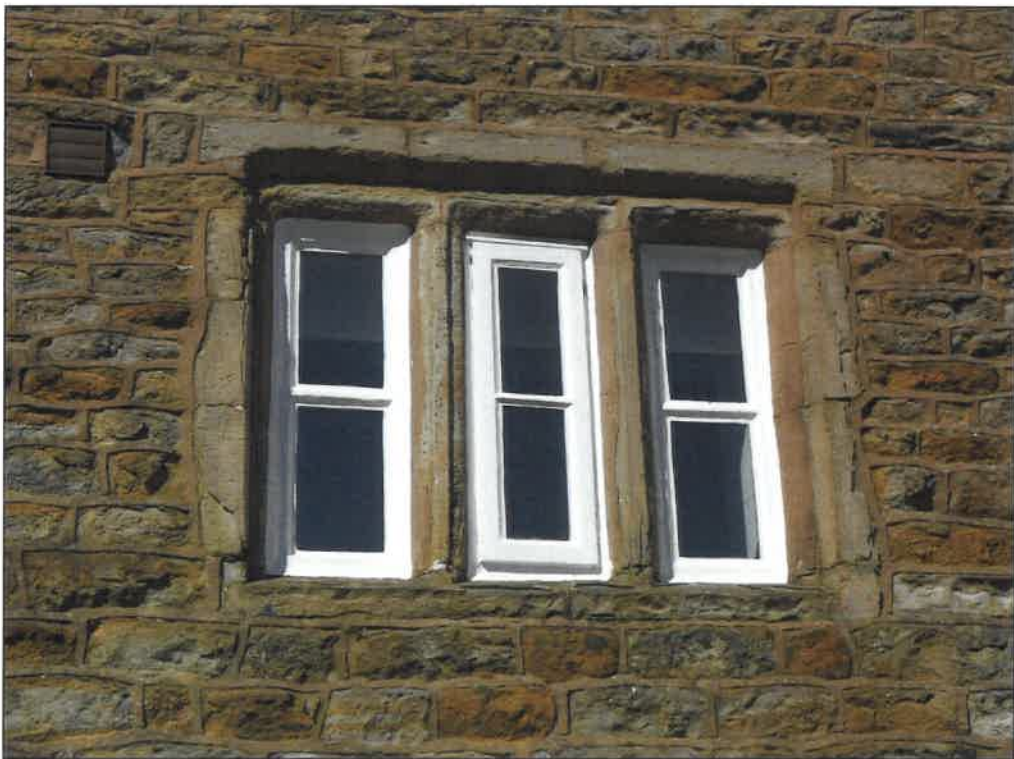
PL11: Window present to the first floor of the rear east facing elevation with ovolo moulded mullions
