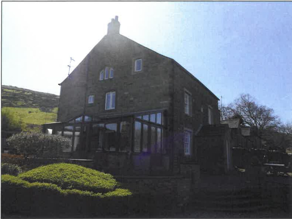
PL02: View of the building from the north west
