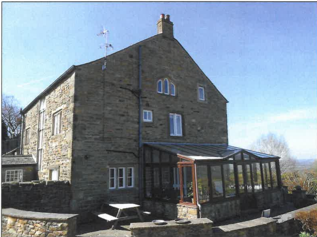
PL03: View of the building from the north
