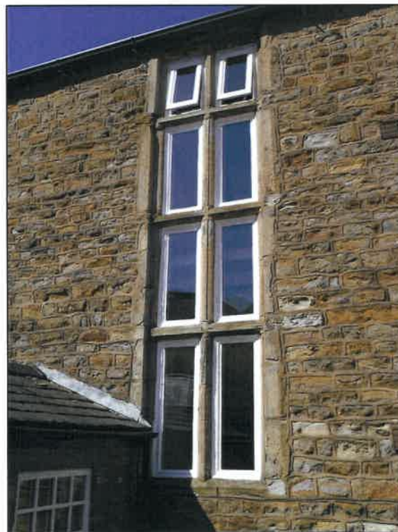
PL09: Existing staircase window present to the rear east facing elevation
