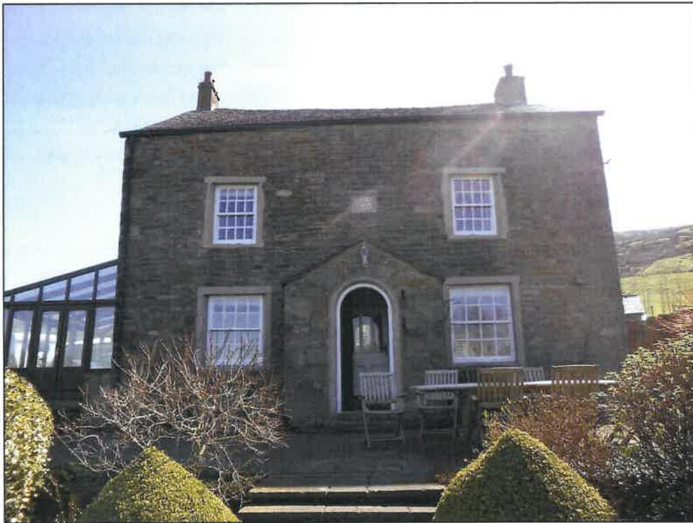
PL01: View of the front of the building from the west
