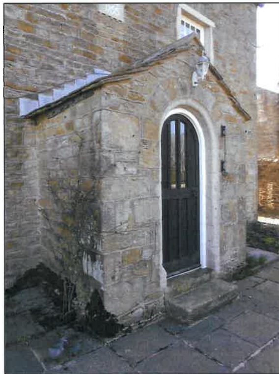
PL05: Front entrance porch to the west elevation of the building
