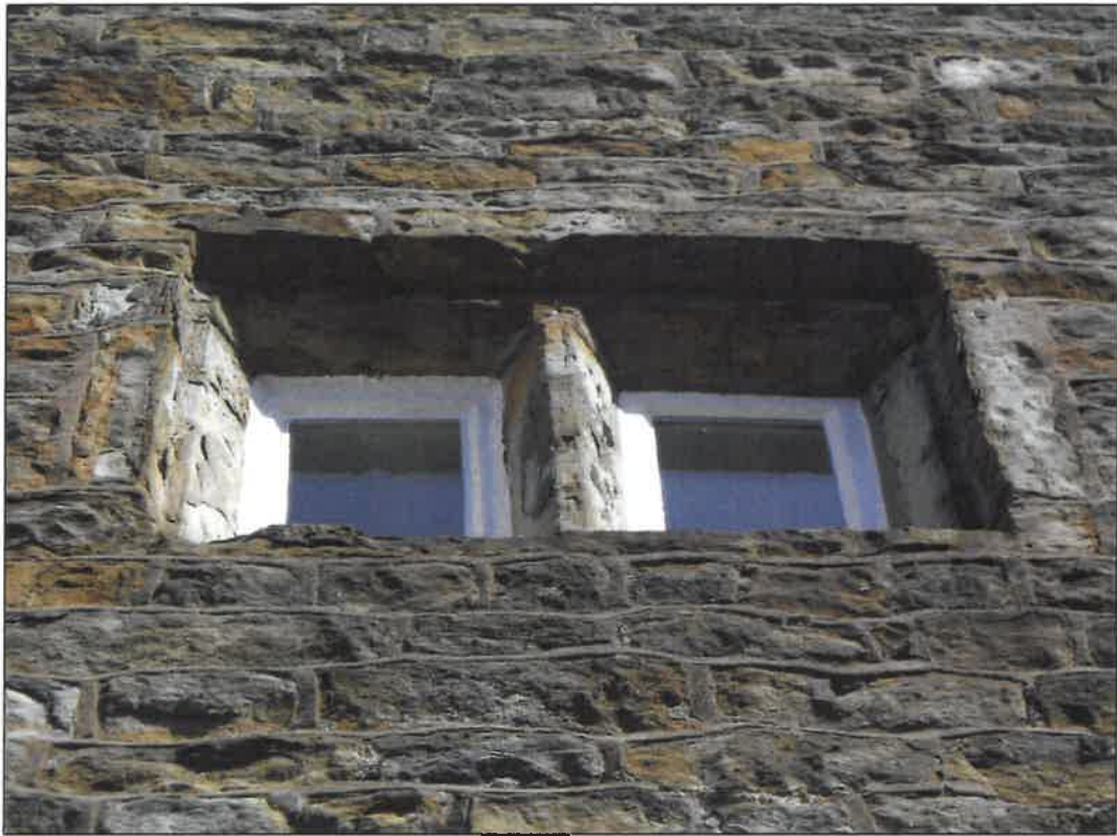
PL10: Window present to the second floor with straight chamfered mullion and jambs.
