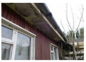
The property has no accessible loft space present, timber soffits and barge boards are present and are close fitting with no obvious crevices or gaps.
