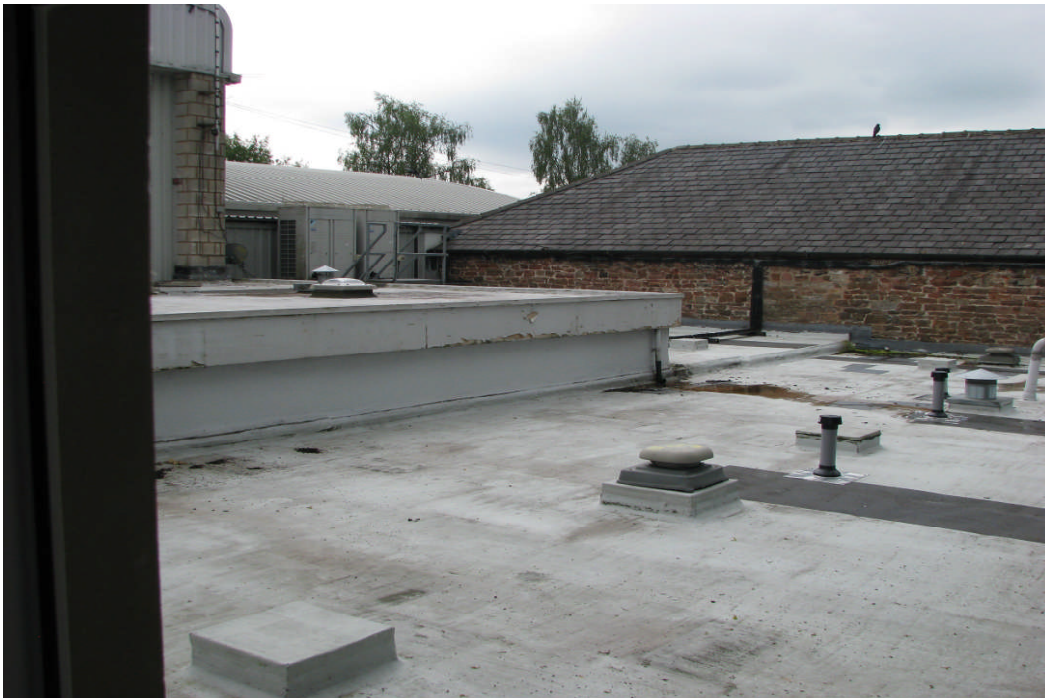
Existing roof area
