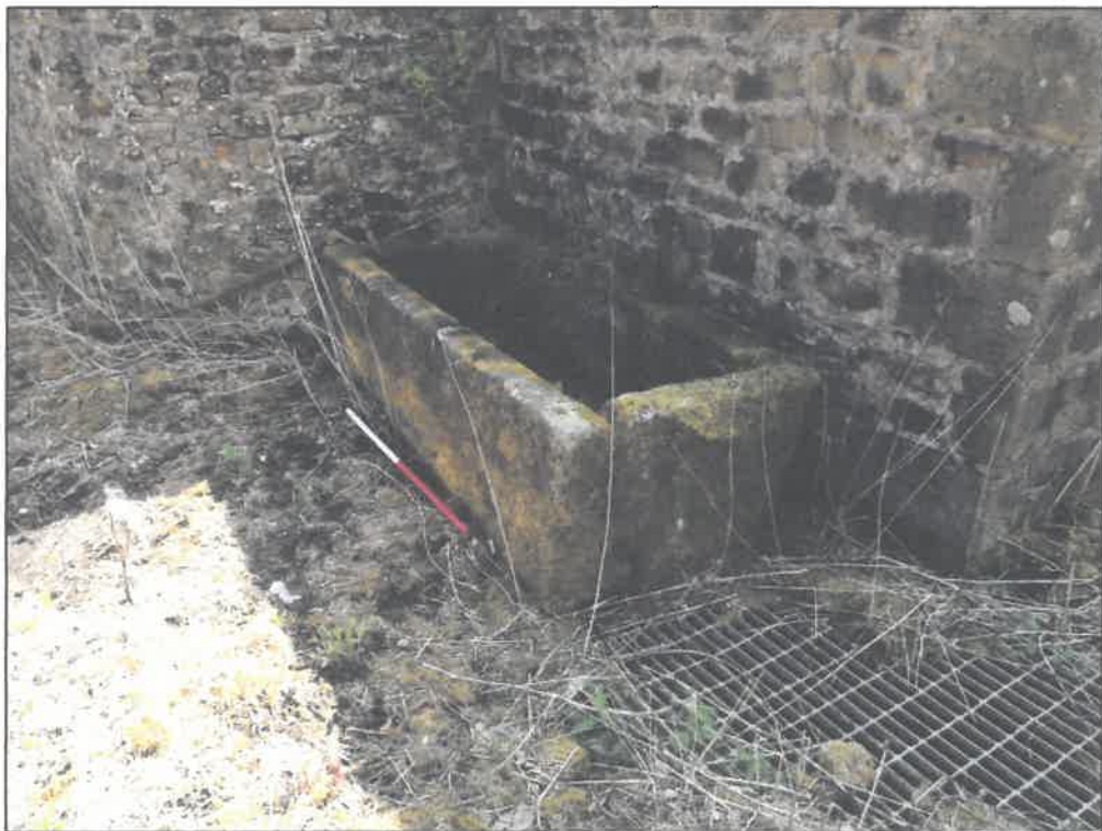
Plate 14. Stone trough and drain, looking north-east, scale 1m
