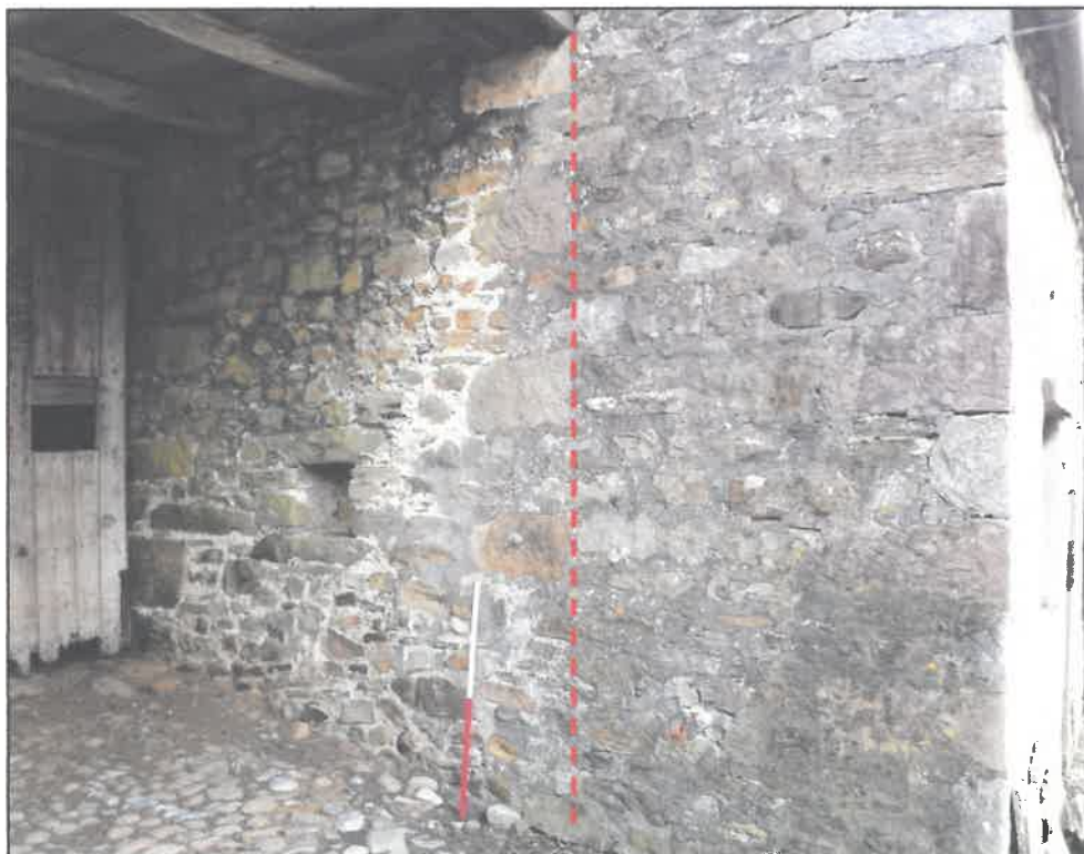
Plate 6. Lantern niche & butt join of Phase II extension, looking NE, scale 1m
