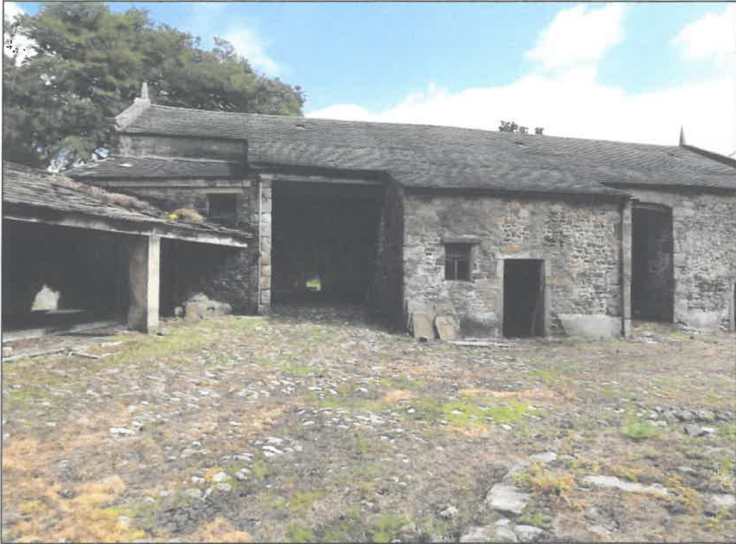
Western end of southern elevation, looking north, scale 1m
