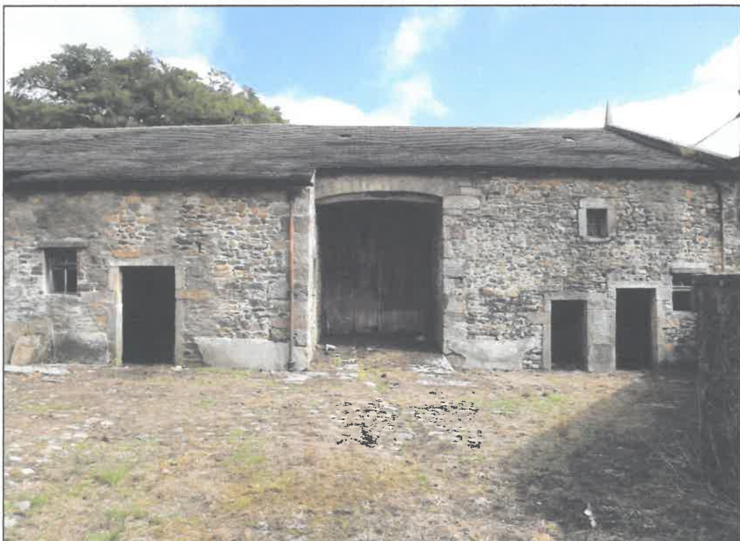
Eastern end of southern elevation, looking north, scale 1m
