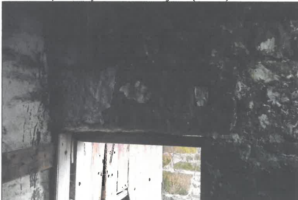
Plate 12. Reused door sill as a jamb, looking east.
