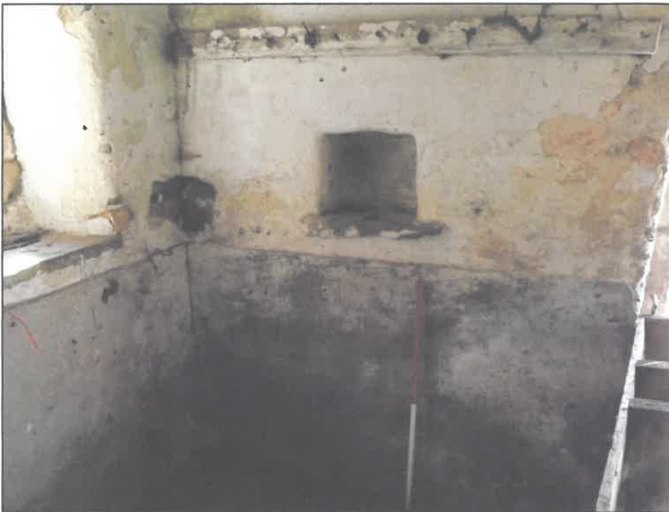
Plate 10. Lantern niche, looking south-east, scale 1m
