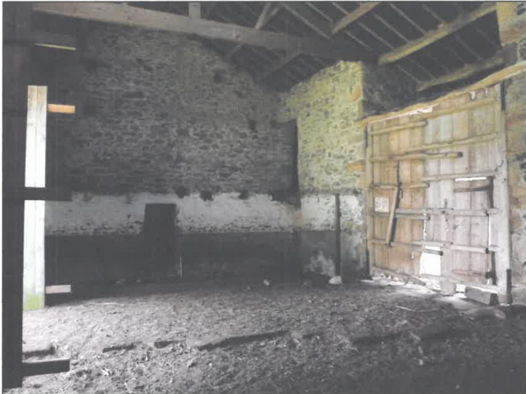
Eastern part of main barn, looking west, scale 1m
