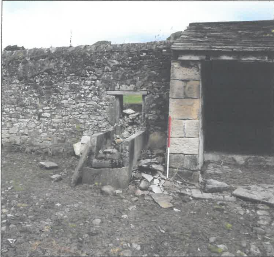
Plate 17. Concrete trough, looking west, scale 1m
