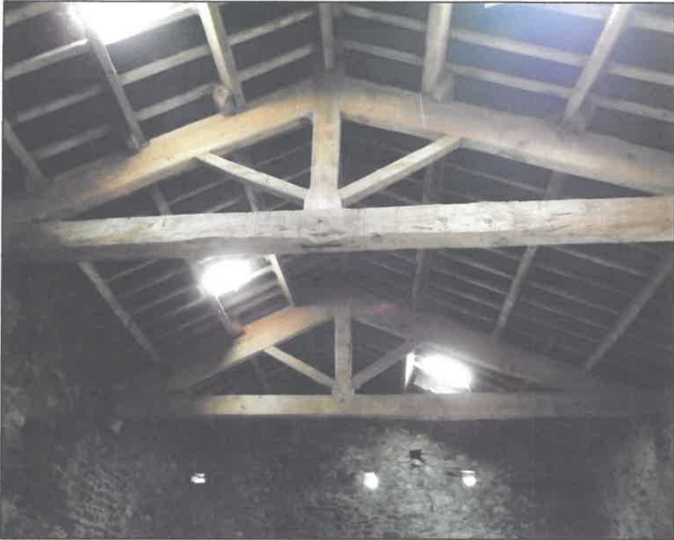
Plate 11. Later trusses at the eastern end of the barn, looking east
