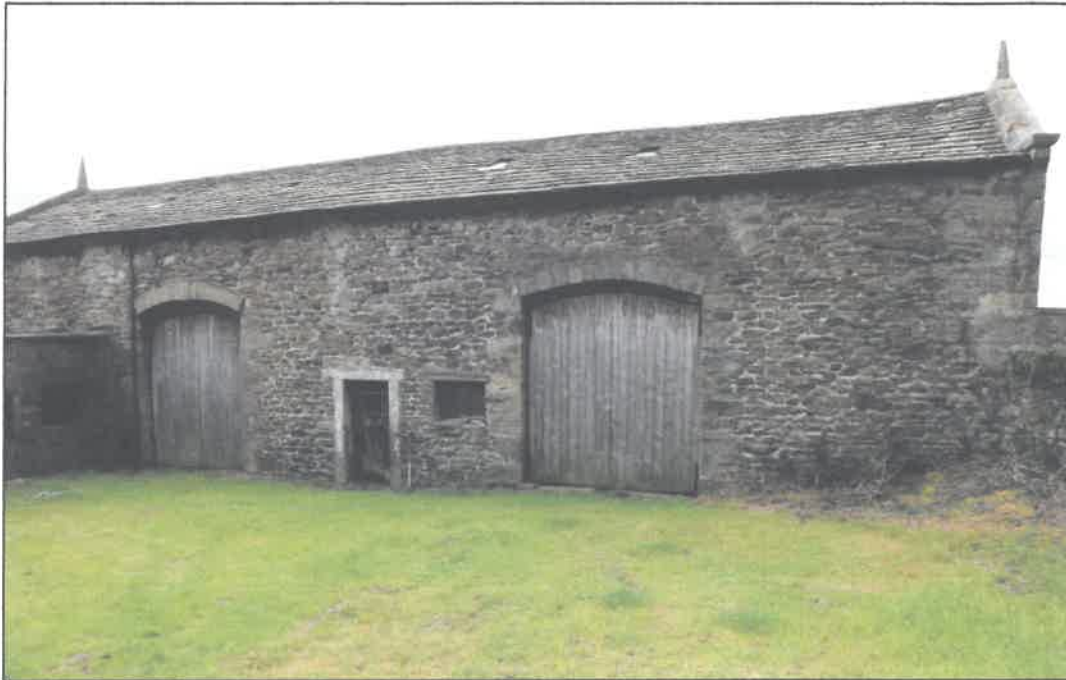
Plate 1. Rear (northern) elevation, looking south, scale 1m
