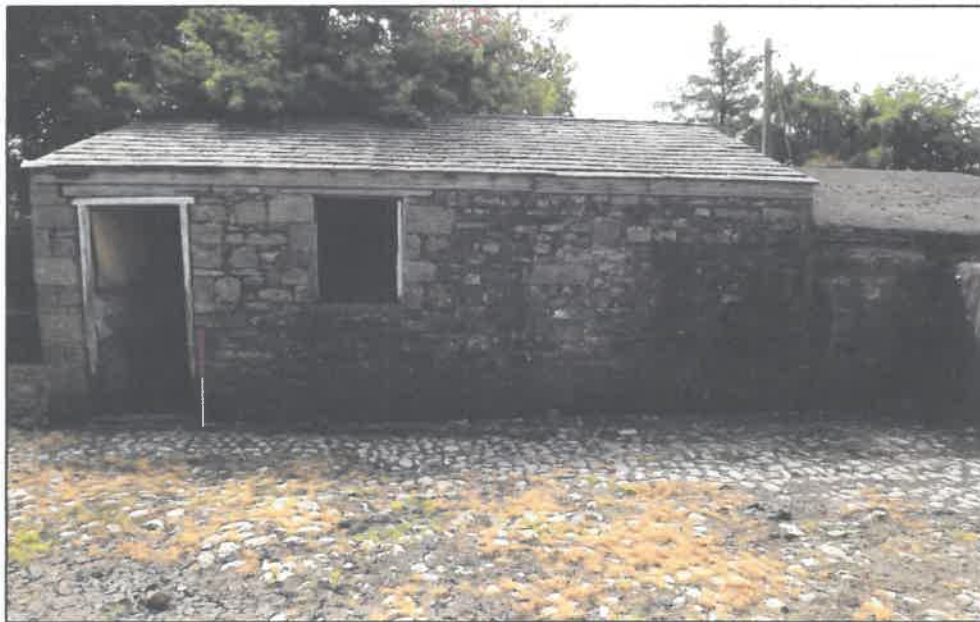
Plate 16. Probable stable, looking east, scale 1m
