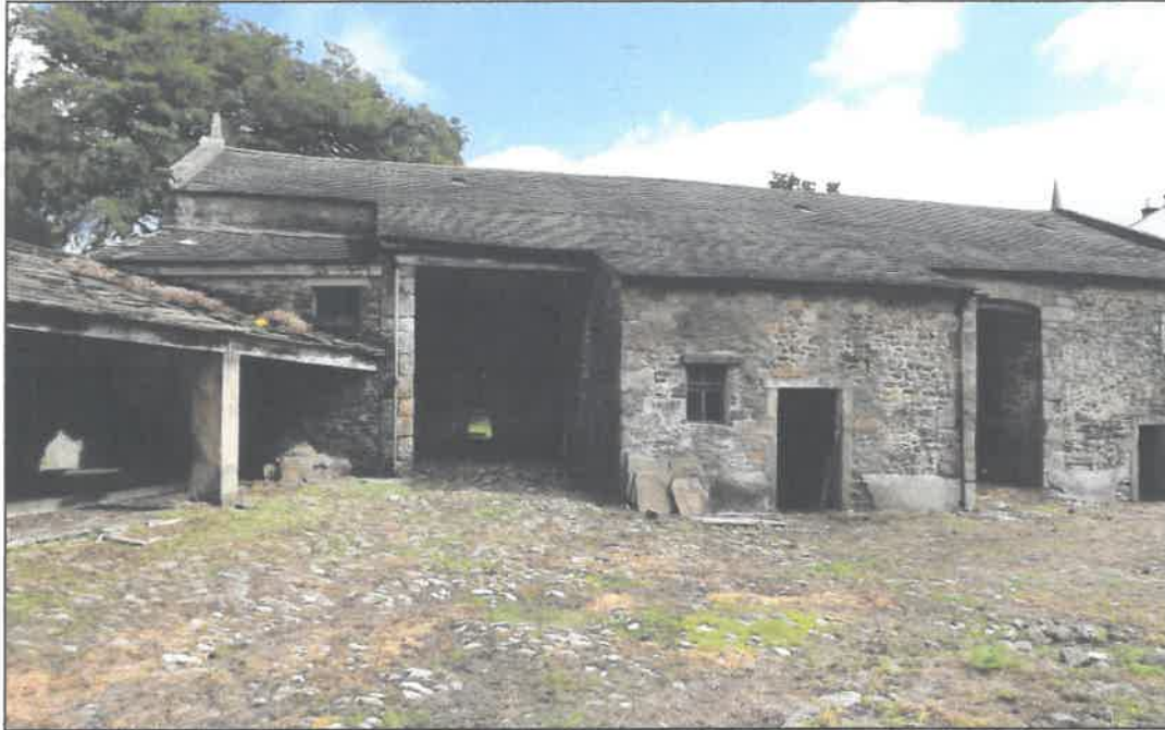
Plate 2. Front (southern) elevation, looking north, scale 1m
