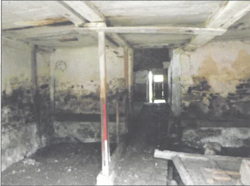
Plate 9. Infill room between porches, looking north, scale 1m
