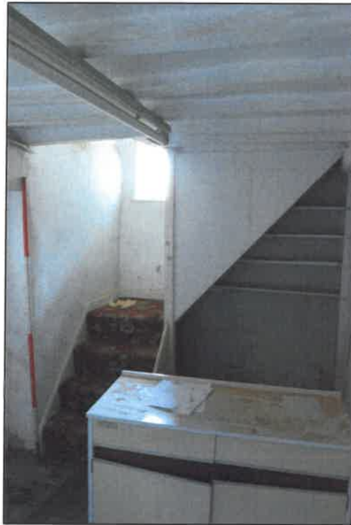
PL08: View east within the north ground floor unit of no.13 Gisburn Road (2m scale).
