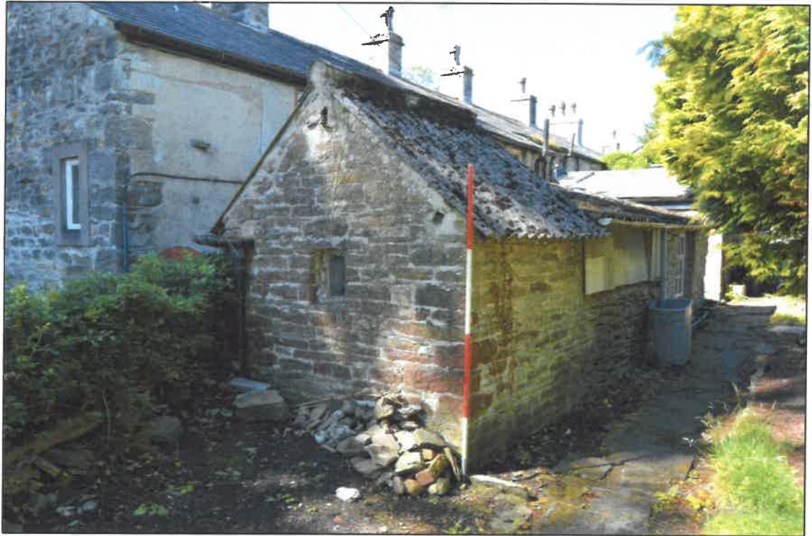
PL04: Outbuilding present to the rear of no.13 Gisburn Road (2m scale).
