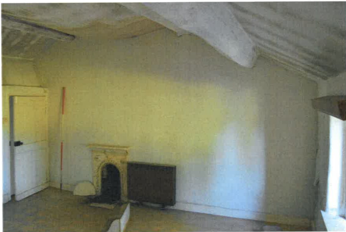
PL12: View east within the first floor south unit of no. 13 Gisburn Road (2m scale).
