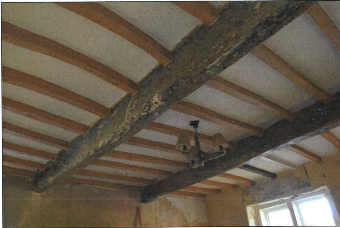
PL06: View of floor structure to the south ground floor unit ceiling to no.13 Gisburn Road.
