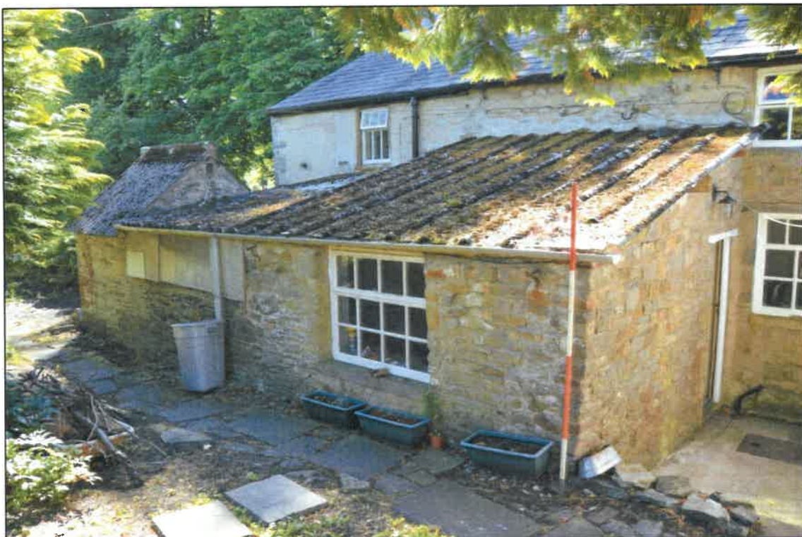
PL03: North facing rear elevation of no's 11 and 13 Gisburn Road (2m scale).
