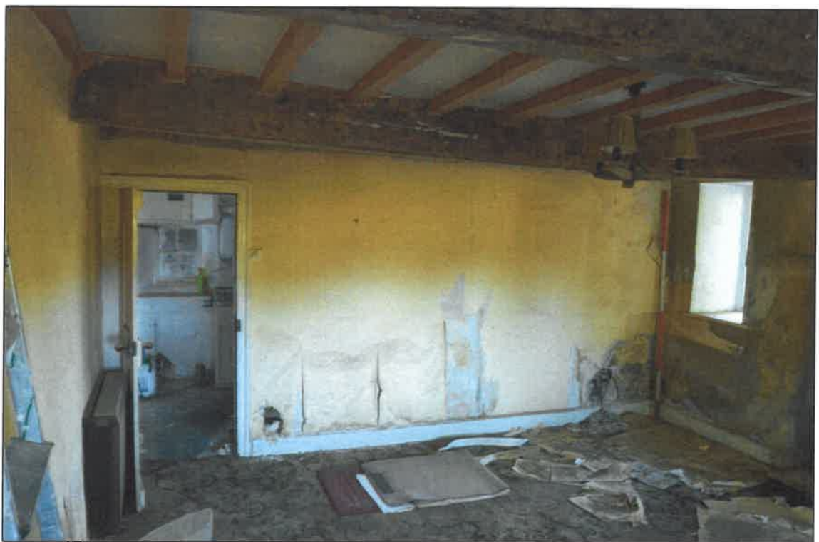
PL05: View north within the ground floor south unit to no.13 Gisburn Road.
