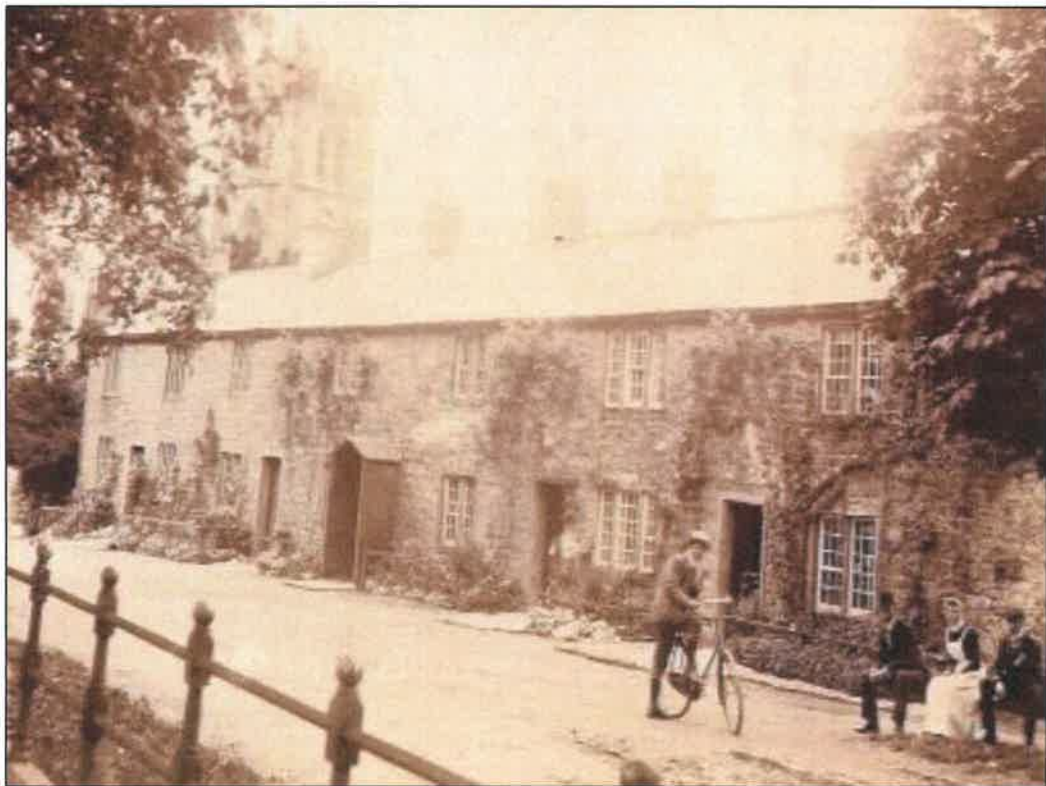
PL18: Photograph showing no's 5 to 13 Gisburn Road in the early 20 th century.
