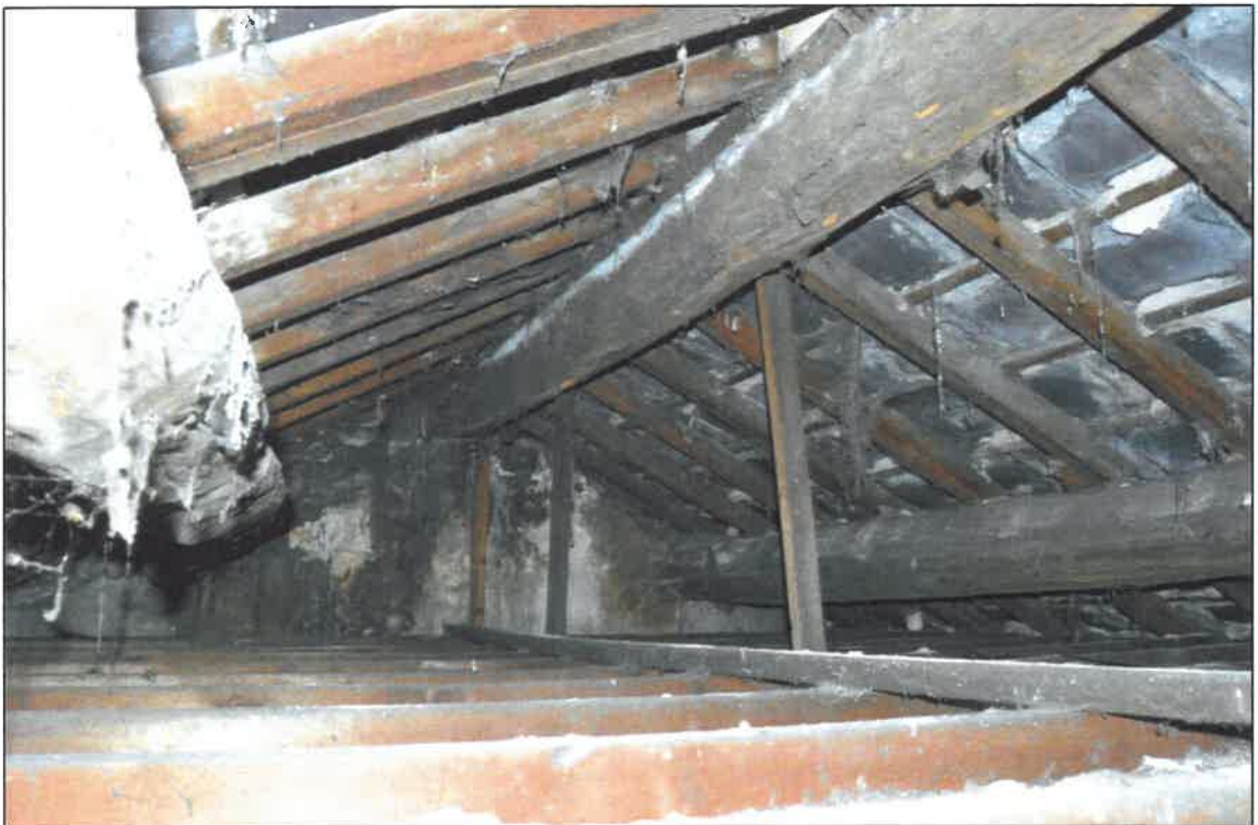
PL14: View of timber roof structure over the south first floor unit of no. 13 Gisburn Road.
