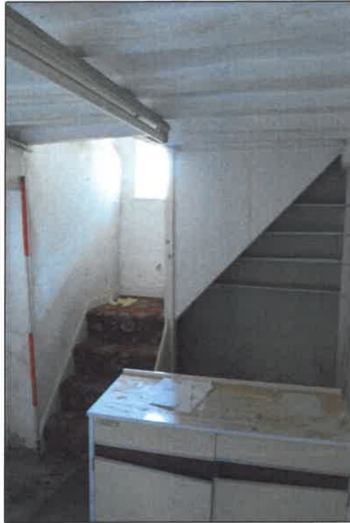
PL08: View east within the north ground floor unit of no. 13 Gisburn Road (2m scale).
