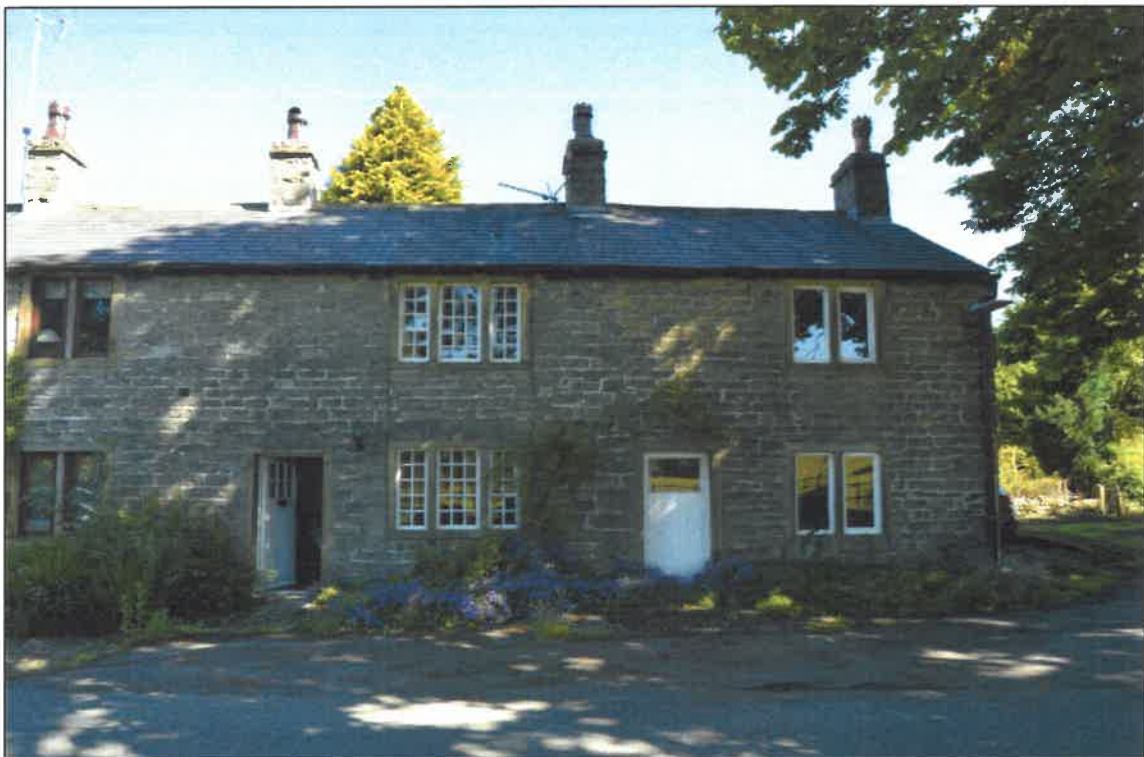
PL01: South facing elevation of no's 11 and 13 Gisburn Road (2m scale).
