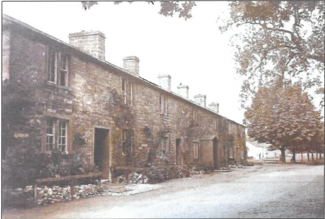
PL19: Photograph showing no's 5 to 13 Gisburn Road in the early 20 th century.
