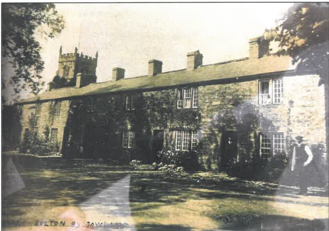
PL20: Photograph showing no's 5 to 13 Gisburn Road in the early 20 th century.
