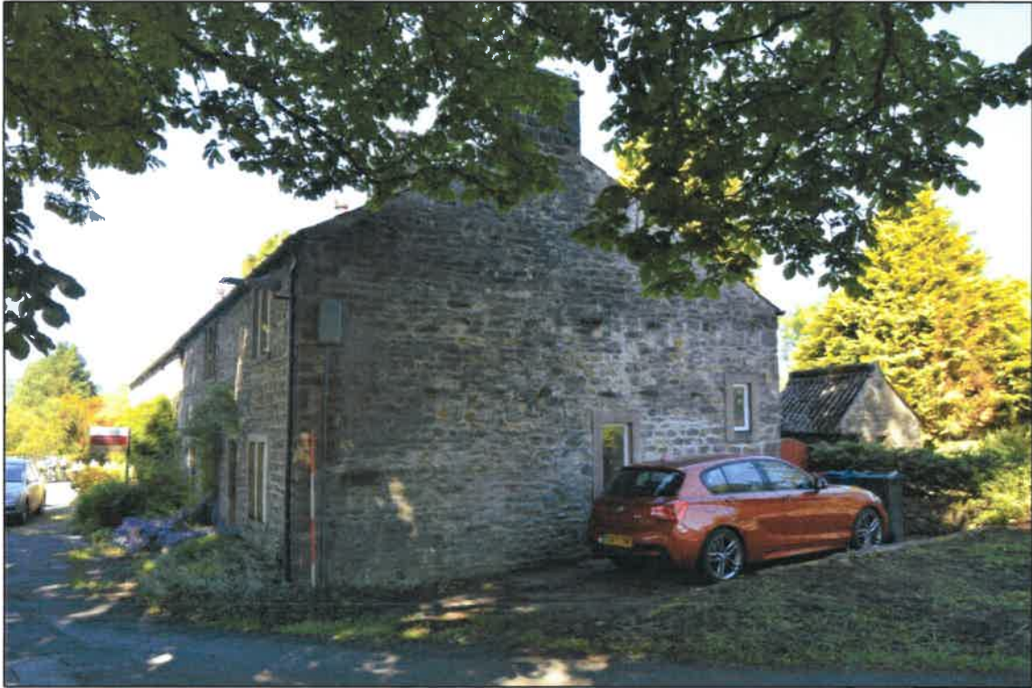
PL02: East facing side elevation of no. 13 Gisburn Road (2m scale).
