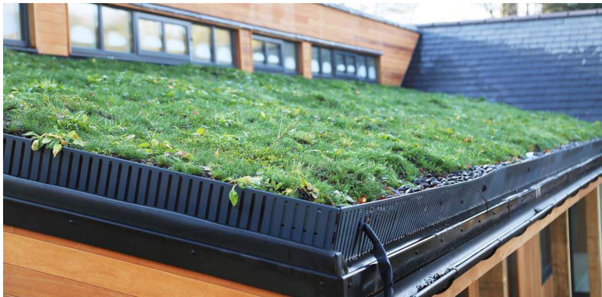
Figure 6.3: Typical Example of a Green Roof
