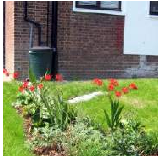
Typical domestic rain garden, Ashby Grove, London | CIRIA
