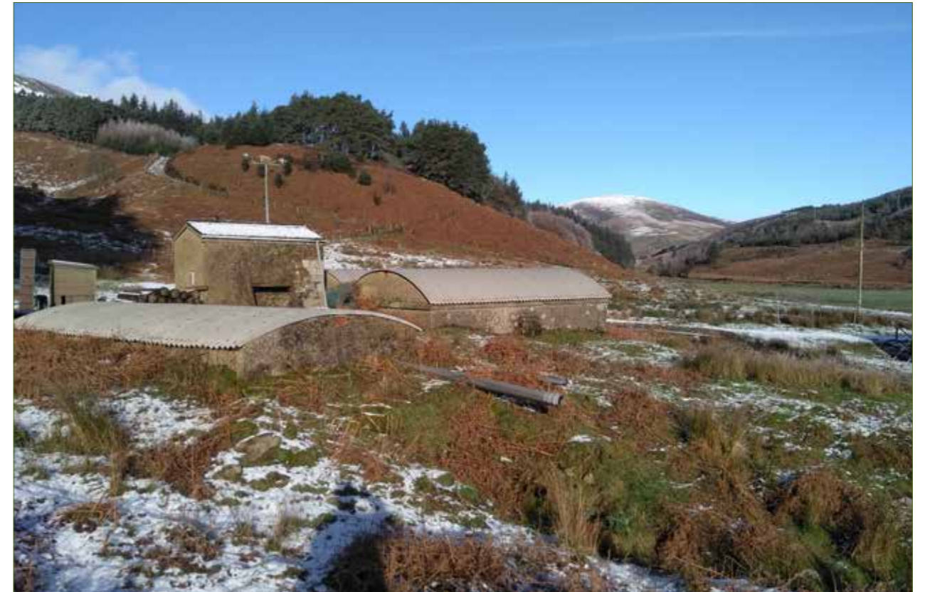
Figure 6 - View of Site showing existing water tank in foreground, with additional outbuildings for conversion / removal.
