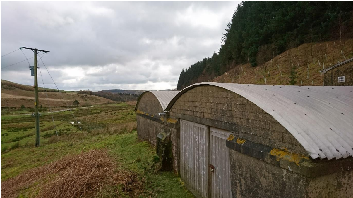
Figure 2: View down the valley, 'tank house' in the foreground, 'plant room' just visible on the right
