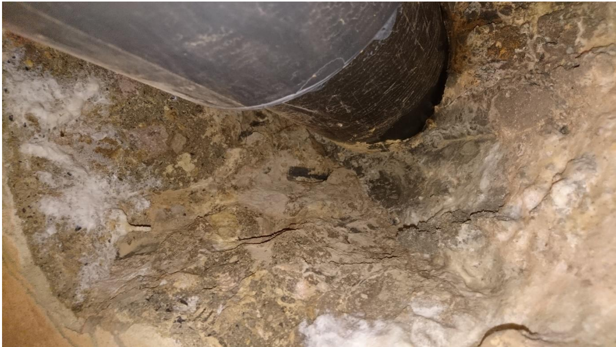
Figure 14: Closeup of opening in rear wall for water supply pipe
