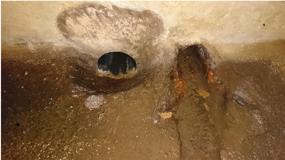
Figure 17: Closeup of drain in front wall
