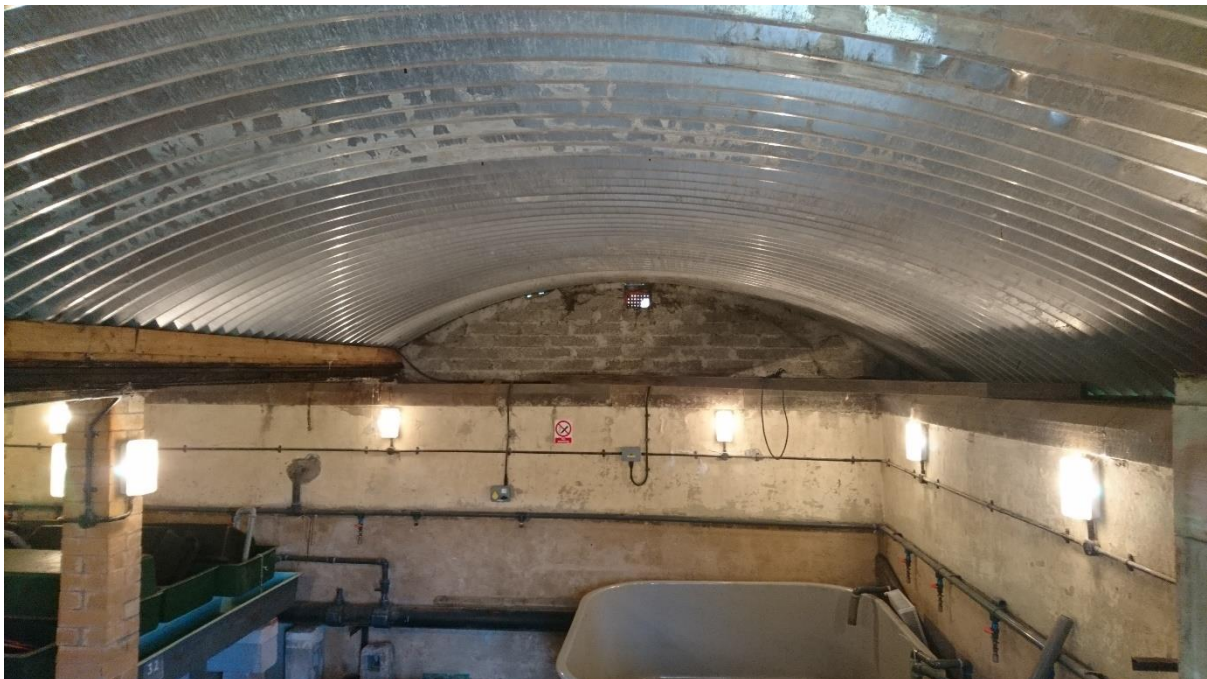
Figure 8: Internal view of tank room steel roof
