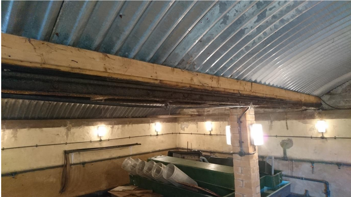
Figure 9: Central girder and supporting pillar
