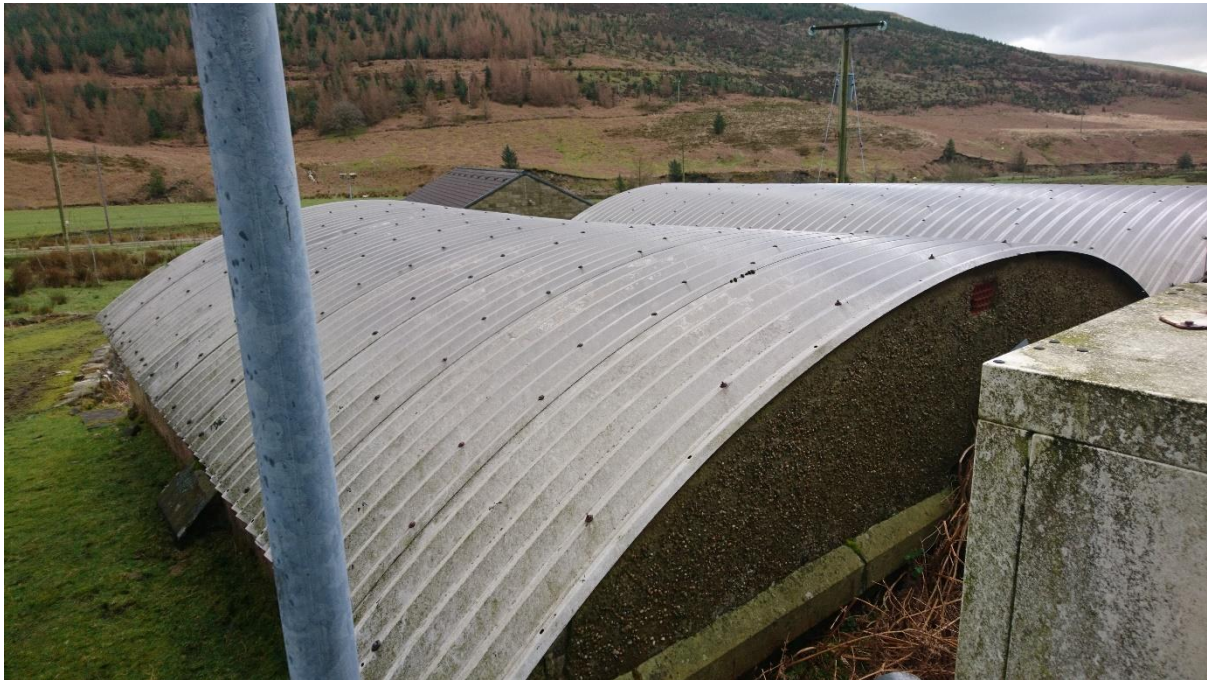
Figure 7: External view of tank room steel roof
