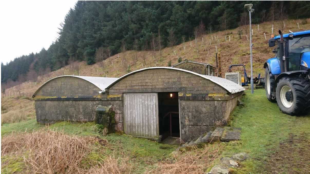
Figure 4: Front (north eastern) elevation of the tank house
