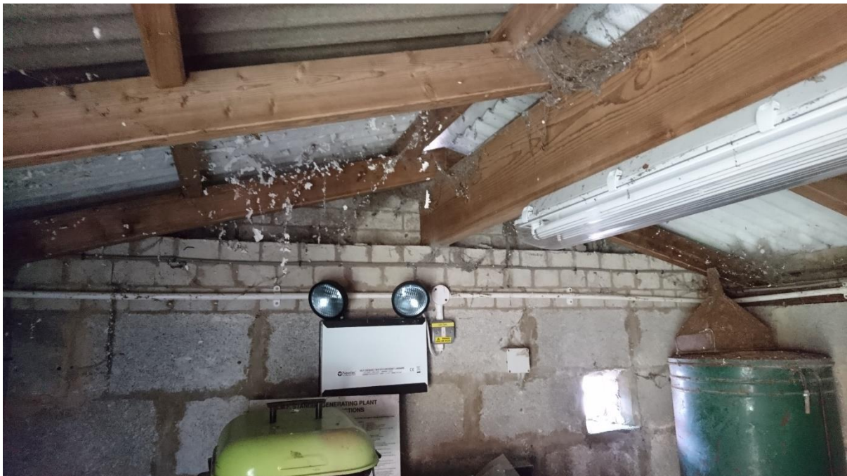
Figure 11: Masonry shelf for ridge beam bearing
