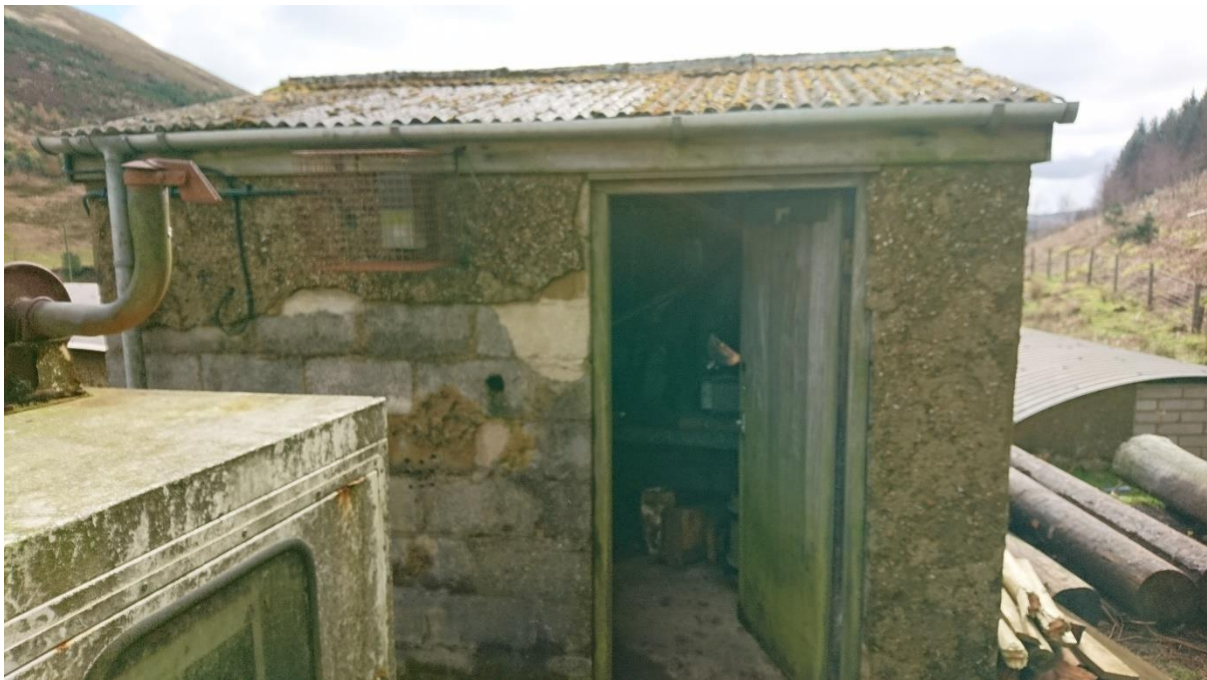
Figure 5: North western elevation of the plant room
