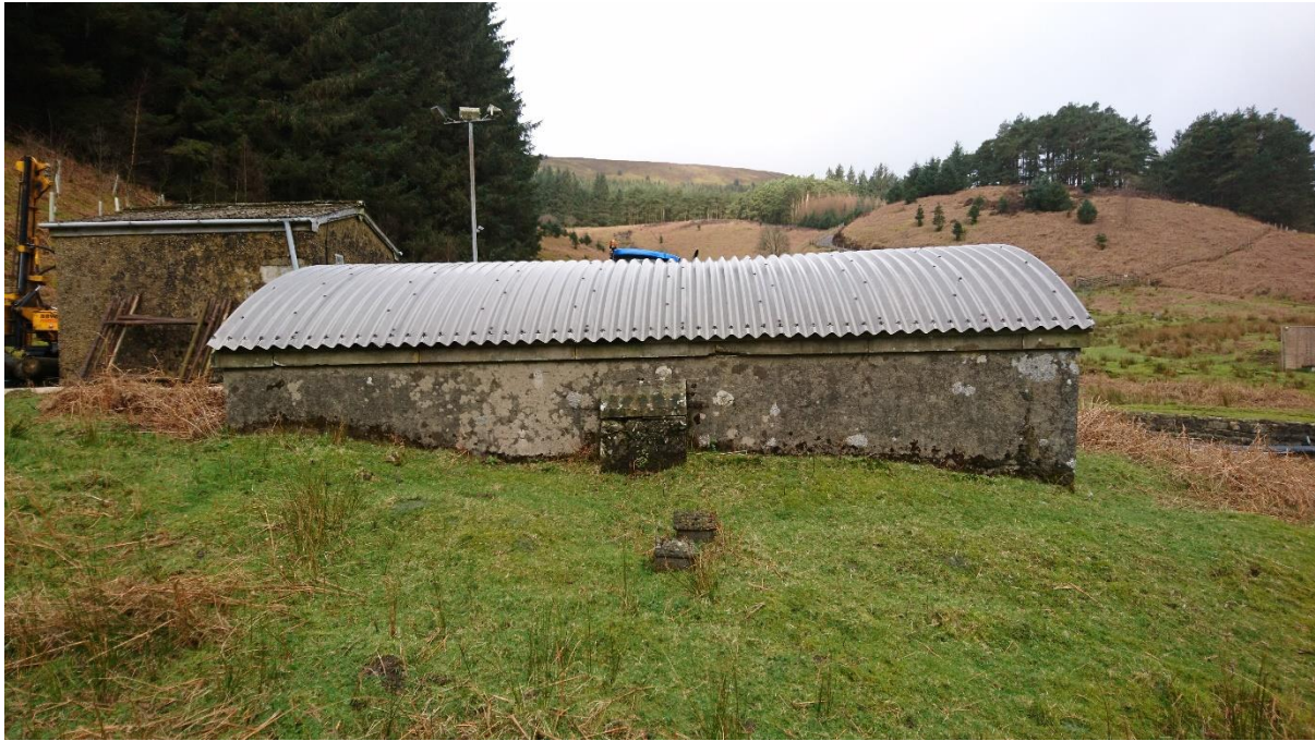
Figure 1: View up the valley, 'tank house' on the right, 'plant room' on the left
