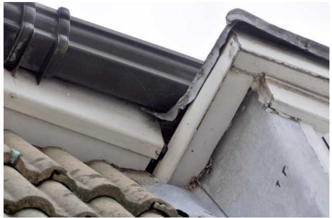
Close up view of gaps associated with soffits (lhs) and gap at join with first floor window (rhs)
