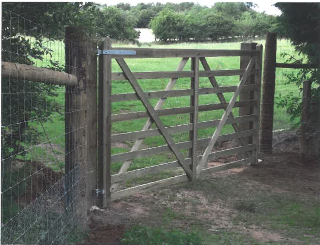
Above is an example of a similar gate that will be used for the dog paddock entrance, with the addition of deer mesh stapled to the gate itself.
