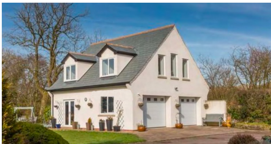
existing views of house and detached outbuilding
