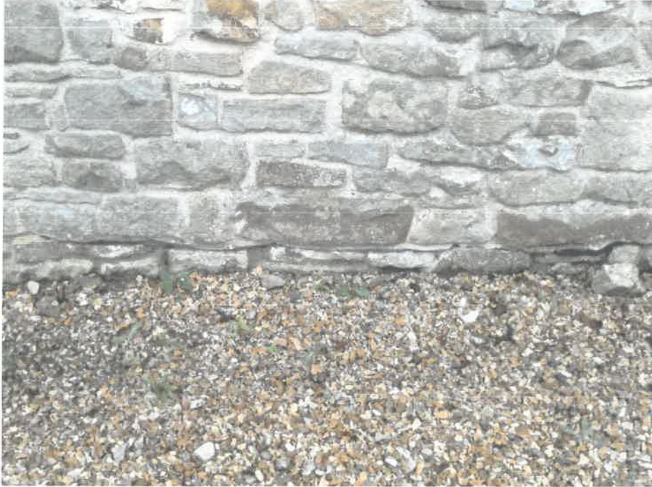
2 : Photo of Dpc in front elevation masonry
