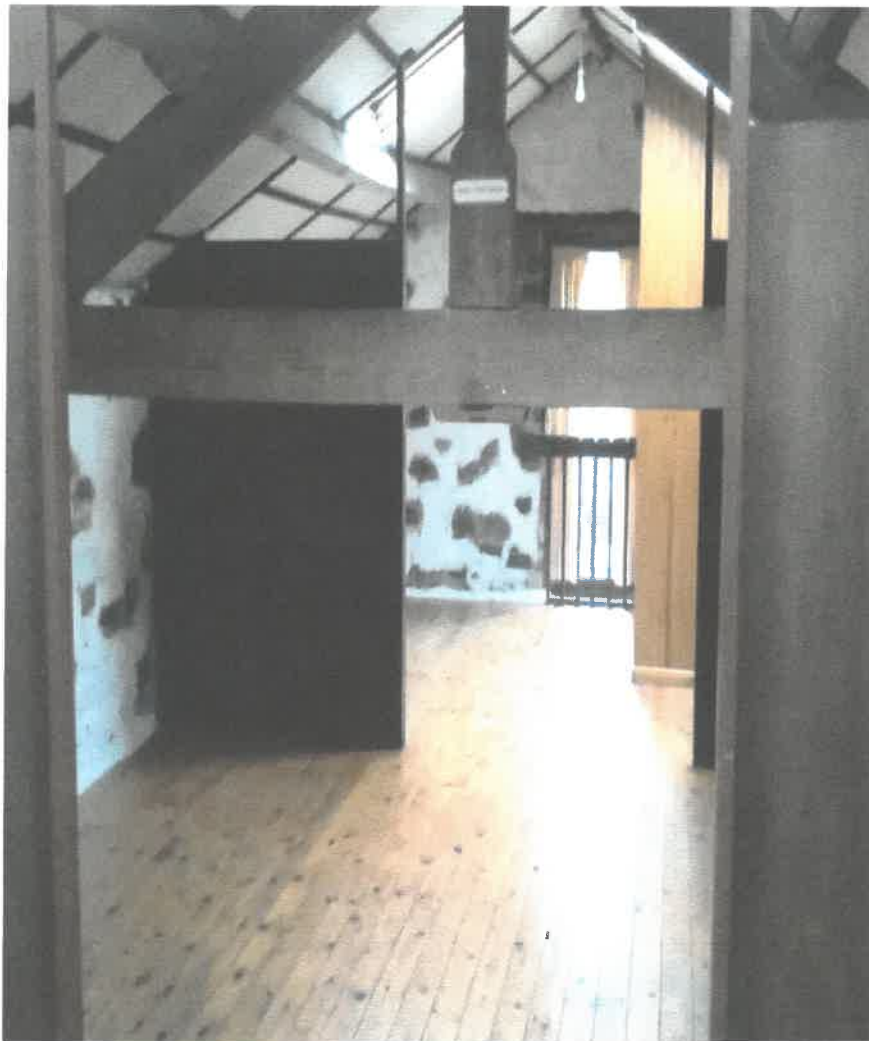
4 : Photo of internal roof structure –
