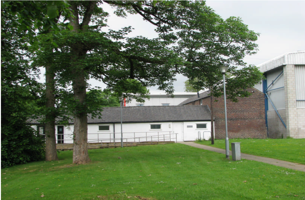
Eastern Elevation showing changing rooms and sports barn gable end
