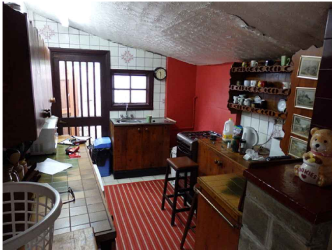
View A - kitchen door and ceiling
