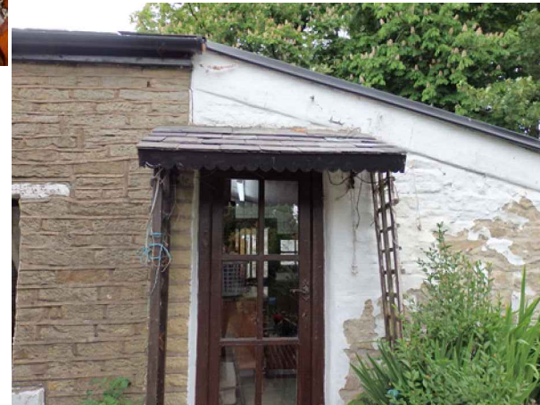
View C - painted outer rear wall
