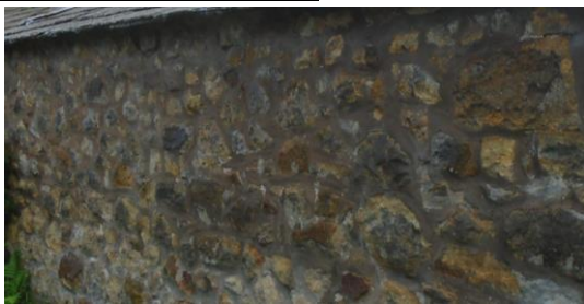
Natural stone walls with flush pointing to the N.W elevation
