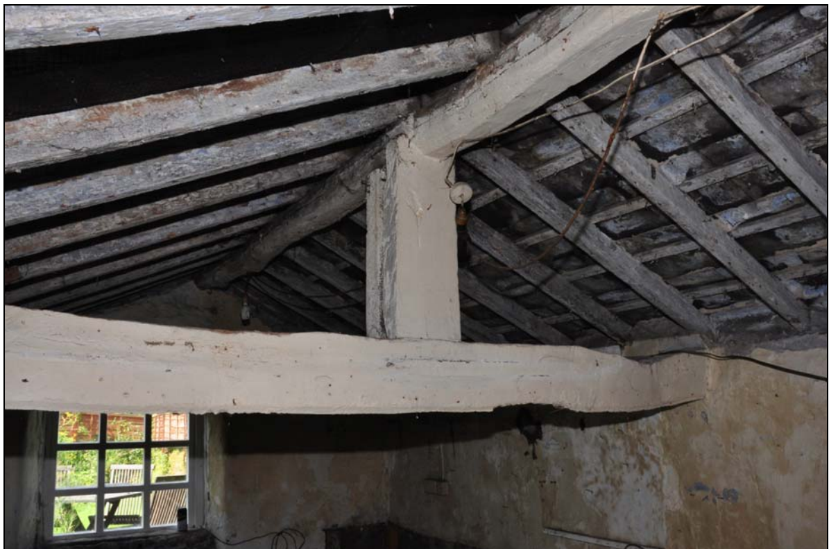
Photo 16: Rear wing: west truss, and other roof members
