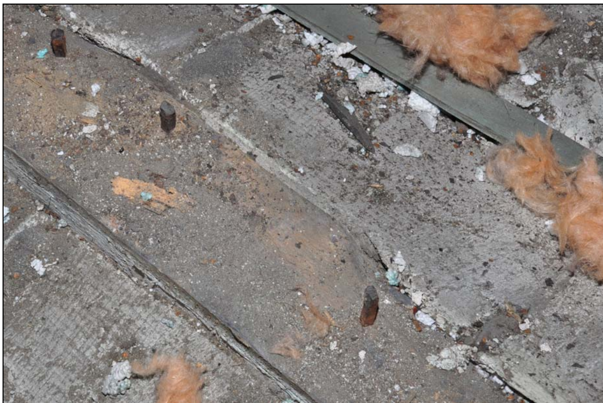
Photo 10: Close-up view of nails for floorboards, in joist on second floor
