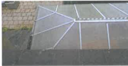
Polycarbonate Conservatory roof
