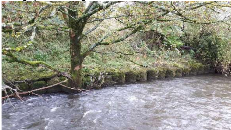
Photograph 4: Hard engineered southern bank of Pendleton Brook
