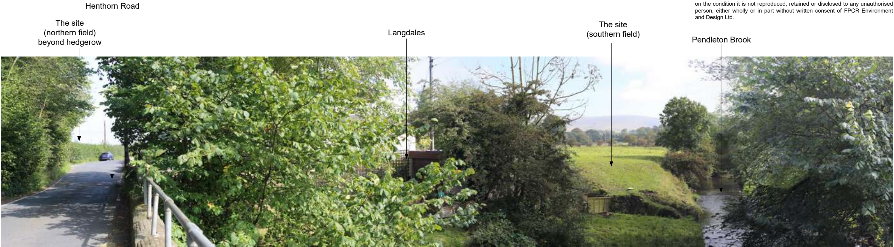
PHOTO VIEWPOINT 8: View east from Henthorn Road (and Ribble Way)
