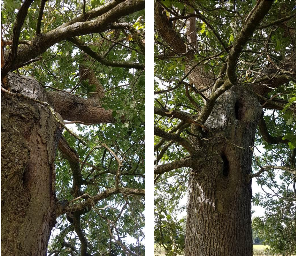
Photographs 3 and 4: Showing further views of visible crack location in north trending limb and entrances to stem cavity
