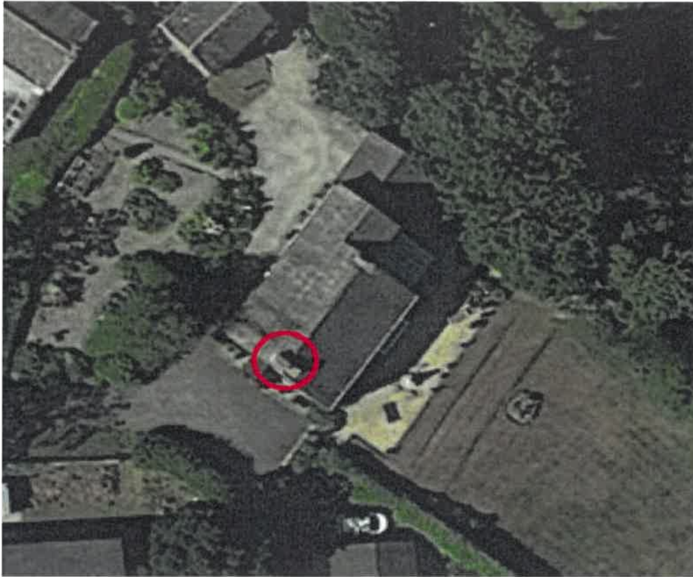
Location of droppings within loft
