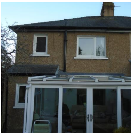
House , lean to and conservatory roofs
