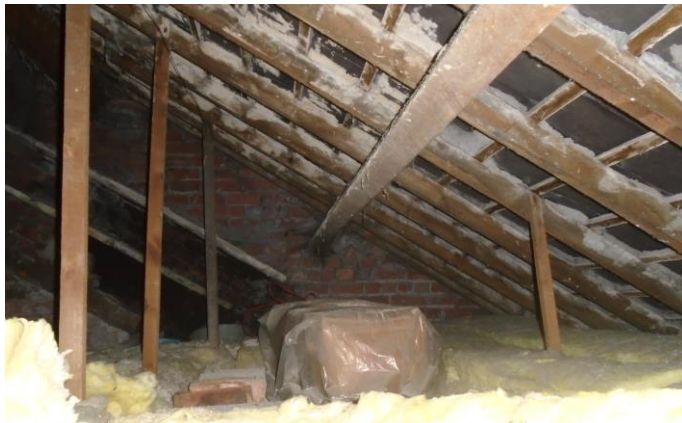
Main roof void
