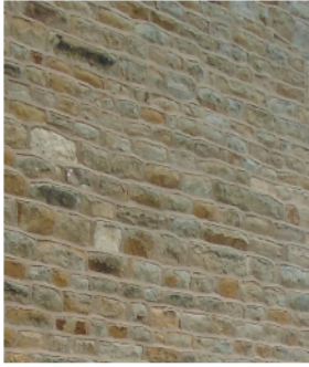
EXTERNAL WALL Natural Stone To Match Existing
