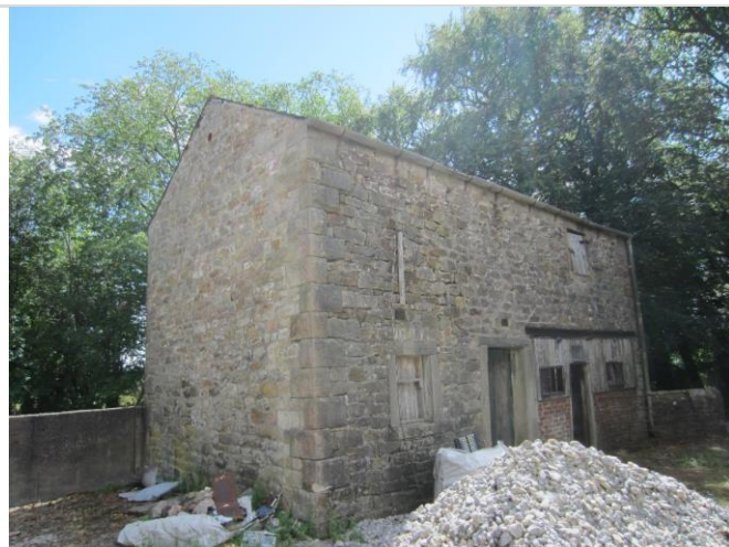
Photo 5: Northern and western elevations of the detached barn
