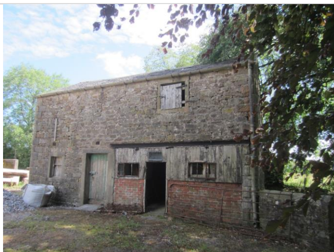
Photo 4: West elevation of the detached barn
