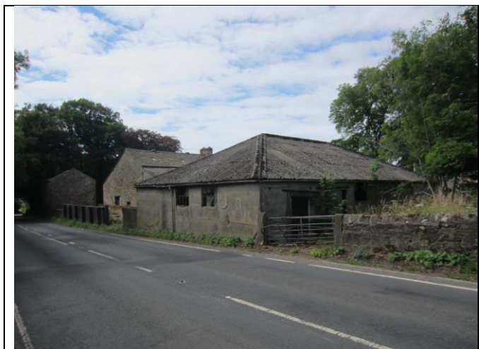
Photo 19: Eastern and northern elevations of the shippon (detached and attached barns in the background)
