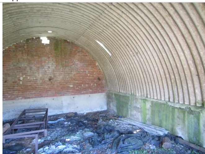
Photo 3: Interior of the nissen hut
