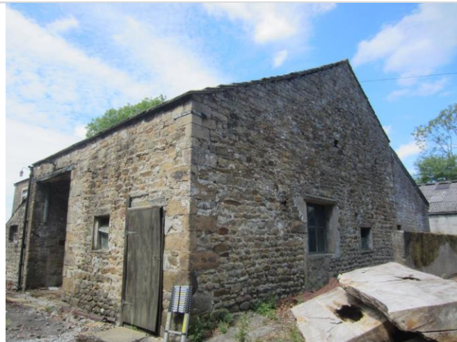
Photo 14: Southern and eastern elevations of the attached barn
