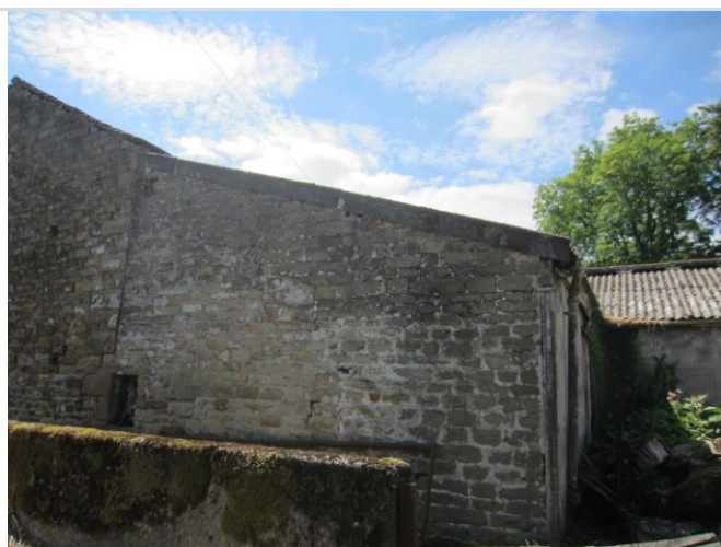
Photo 15: Cement sheet fascia at the eastern elevation of the monopitch / lean-to at the northern elevation of the attached barn
