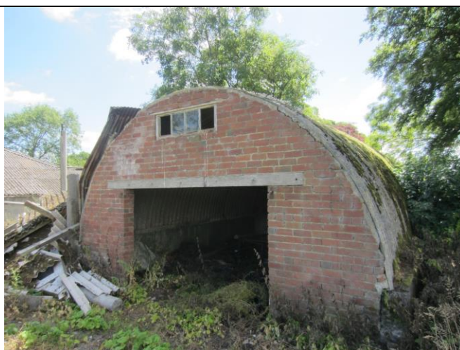
Photo 2: Northern elevation of the nissen hut
