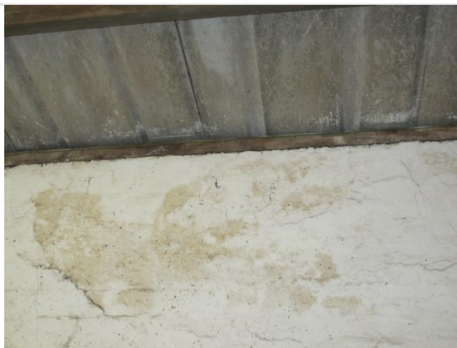
Photo 22: Interior of the shippon showing the timber plank at the wall top
