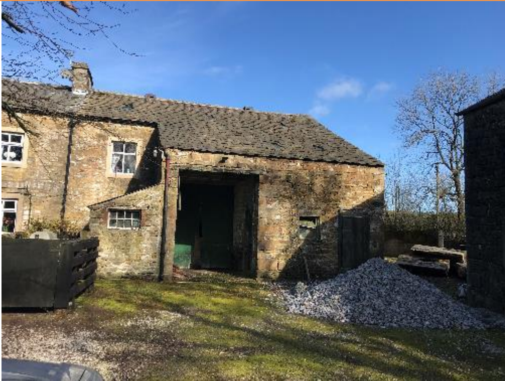
PLATE 3 – VIEW OF THE ADJOINING BARN LOOKING NORTH
