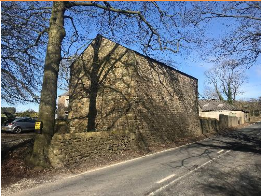
PLATE 2 – VIEW OF THE EASTERN ELEVATION OF THE STANDALONE BARN
