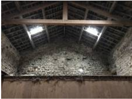
Main barn, walls
