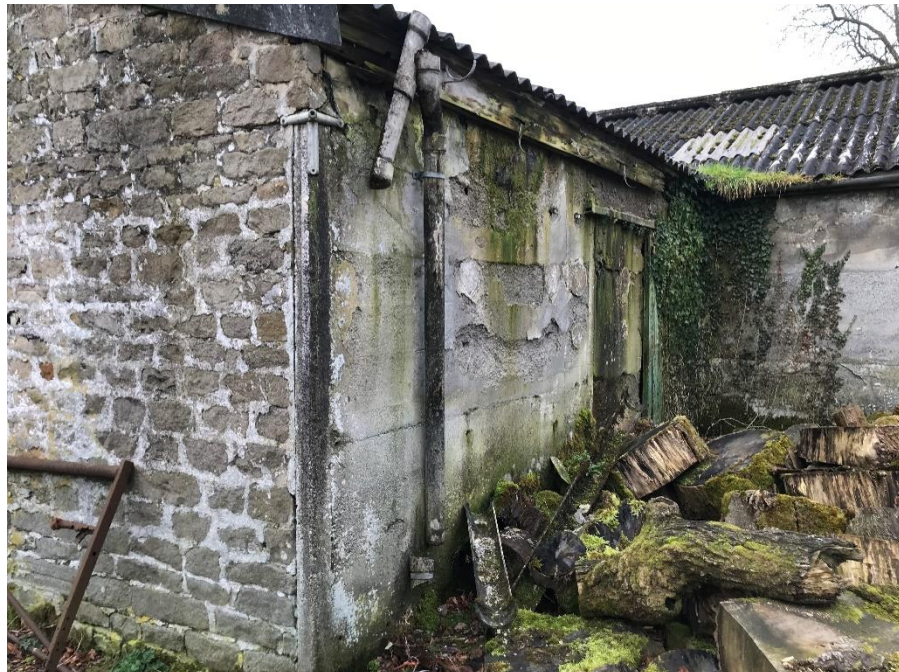
4) North elevation of "lean-to"
