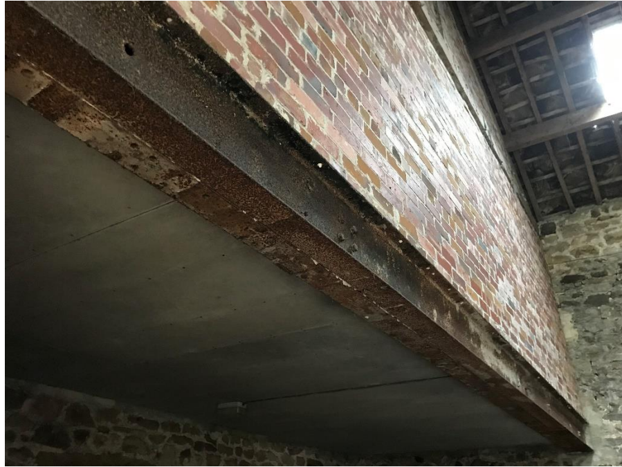
5) Beams spanning across barn supporting party wall and P C planks
