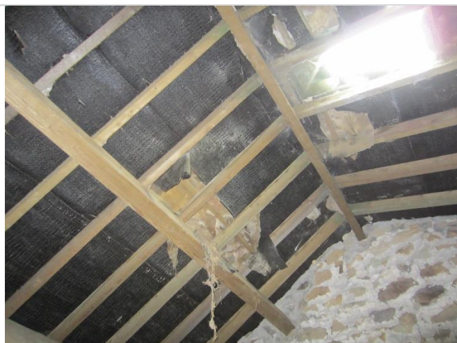
Photo 17: Degraded undertile felt beneath stone tiles at eastern section of the barn (and skylight to create light internal areas)
