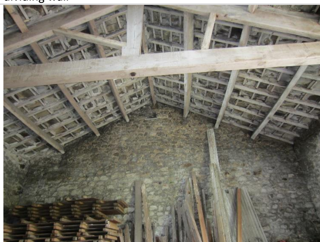
Photo 15: Roof and timbers above single storey / western section of barn
