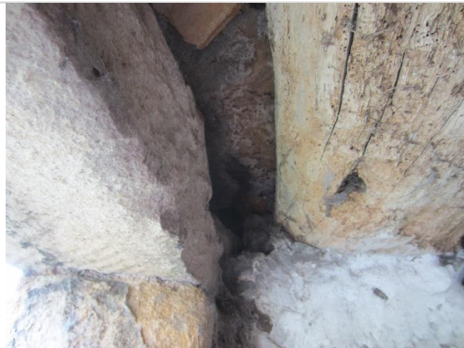
Photo 12: Gaps at timber lintel over doorway on the eastern elevation
