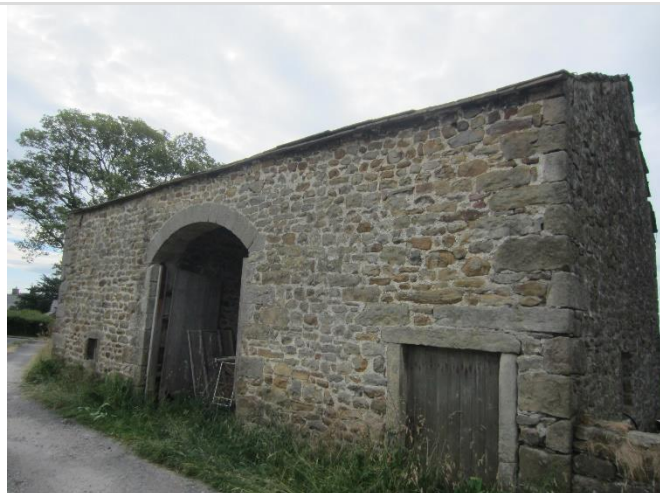
Photo 5: Northern elevation of barn
