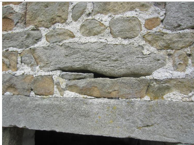
Photo 9: Gaps and PRF at the stone and rubble filled elevation walls (all elevations)
