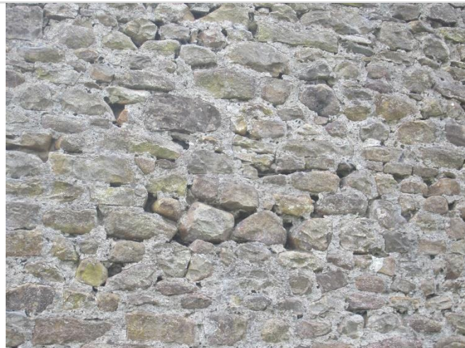
Photo 8: Gaps and PRF at the stone and rubble filled elevation walls (all elevations)
