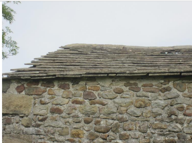
Photo 7: Gaps and PRF between the roof tiles and at the wall tops
