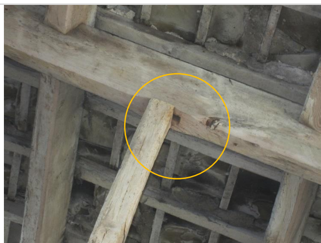
Photo 16: Gaps at mortise joints; no bat present on survey dates
