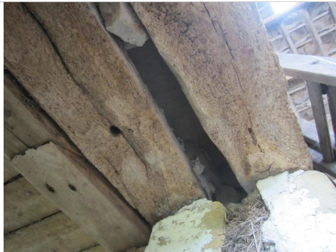
Photo 13: Gaps at timber lintel over doorway at internal dividing wall
