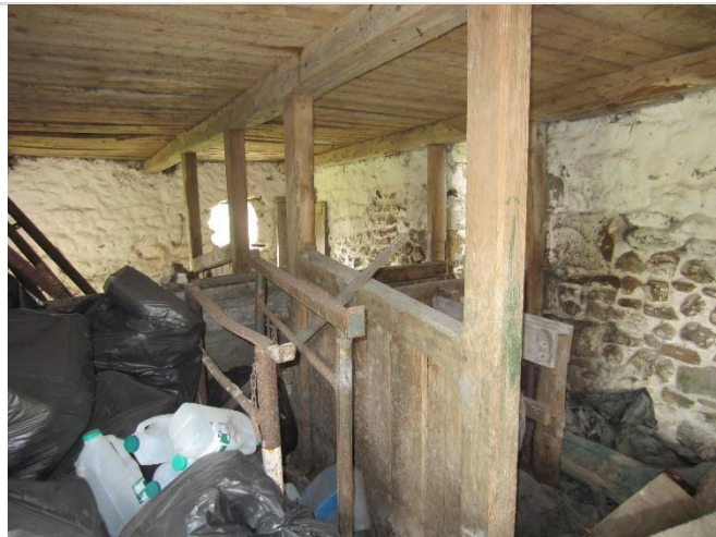
Photo 11: Interior of the eastern section (beneath the hayloft) showing white washed walls
