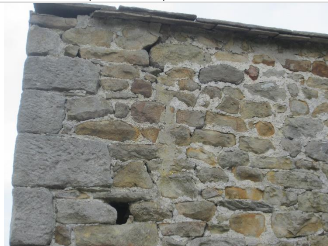
Photo 10: Gaps and PRF at the stone and rubble filled elevation walls (all elevations)
