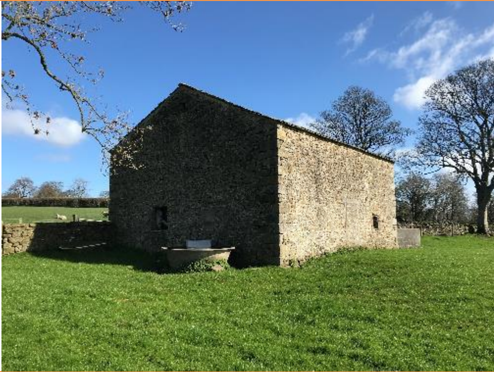
PLATE 3 – VIEW OF THE BARN LOOKING NORTHEAST
