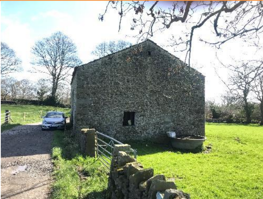
PLATE 1 – VIEW OF THE WESTERN ELEVATION
