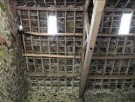
Roof structure, over main space
