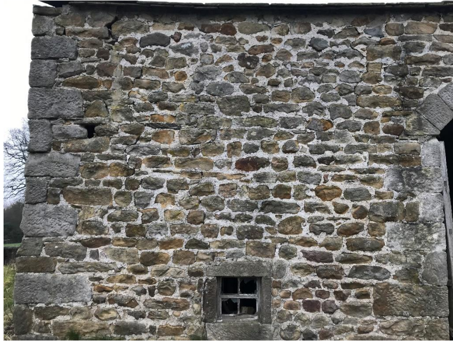
3) Some open joints and discontinuity to adjacent corner
