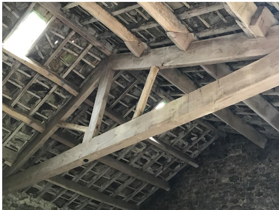
6) Timber roof truss
