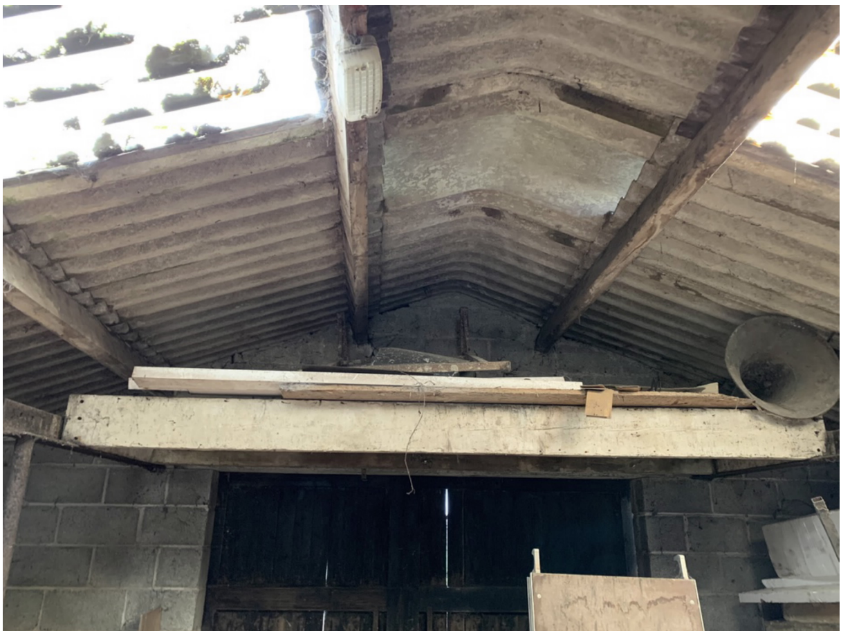
Photo 14 - Internal east end
