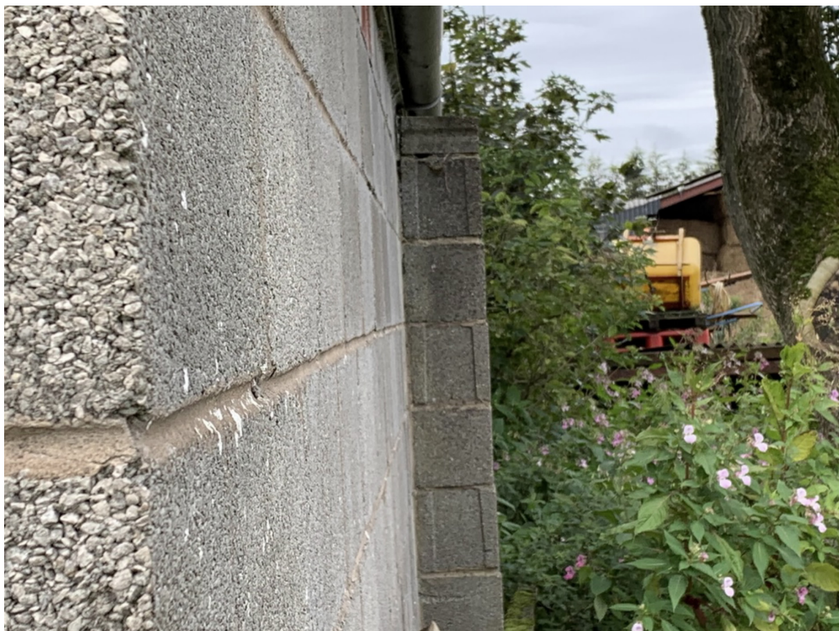
Photo 8 – North Elevation – pier/buttress
