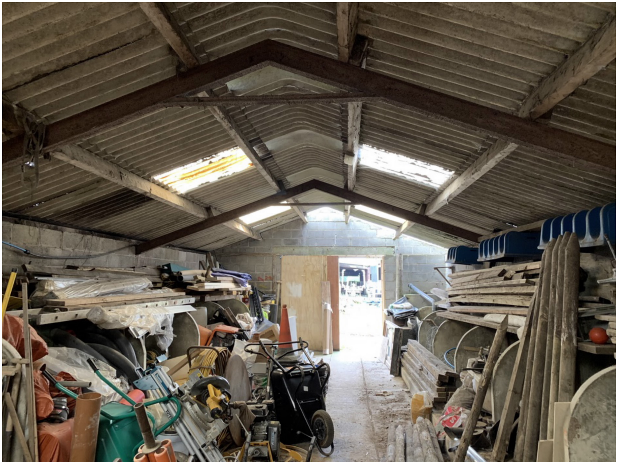
Photo 13 – Internal looking west
