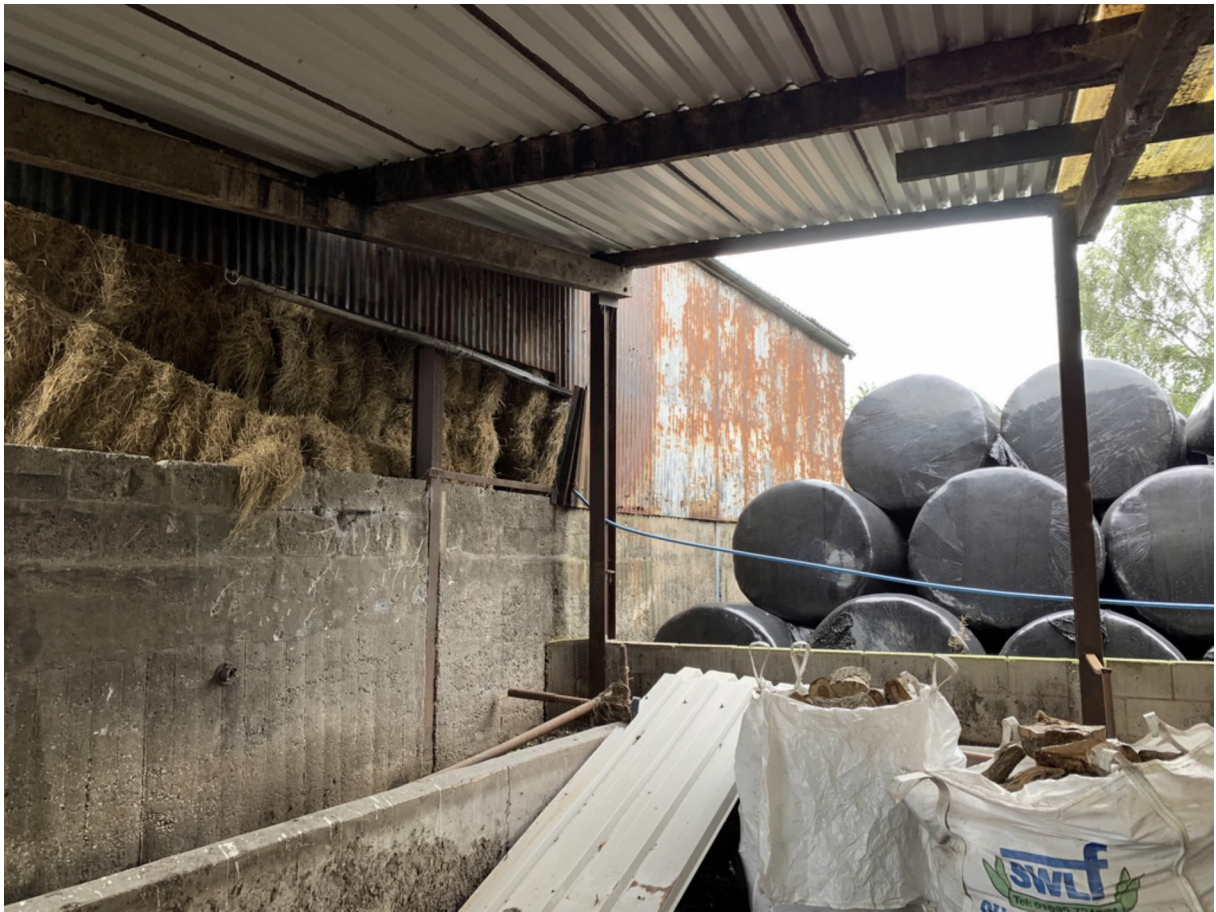
Photo 13 – West Elevation at Rear (north)
