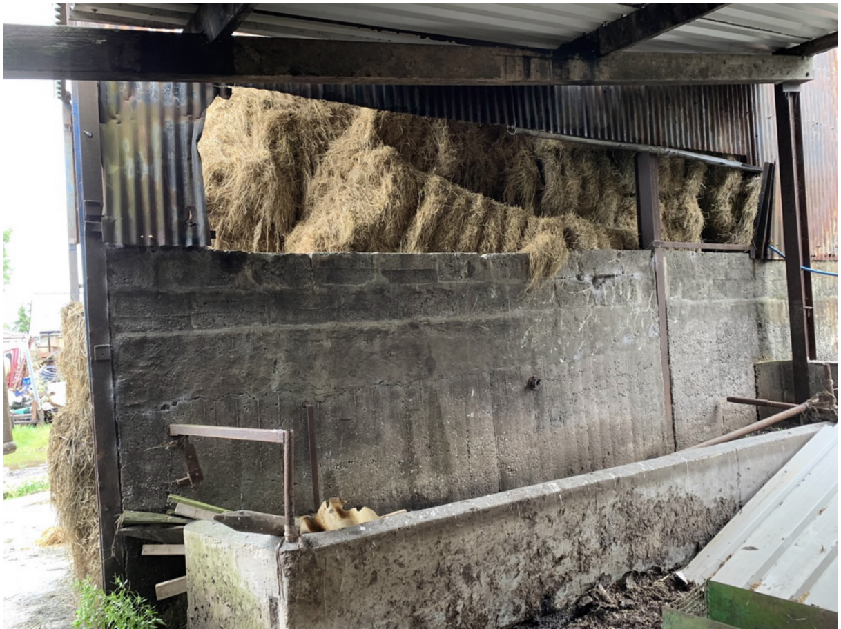
Photo 15 - West Elevation at rear (north)
