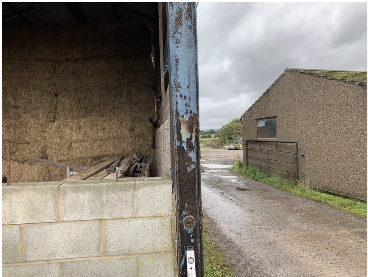
Photo 3- South Gable – Corner Column
