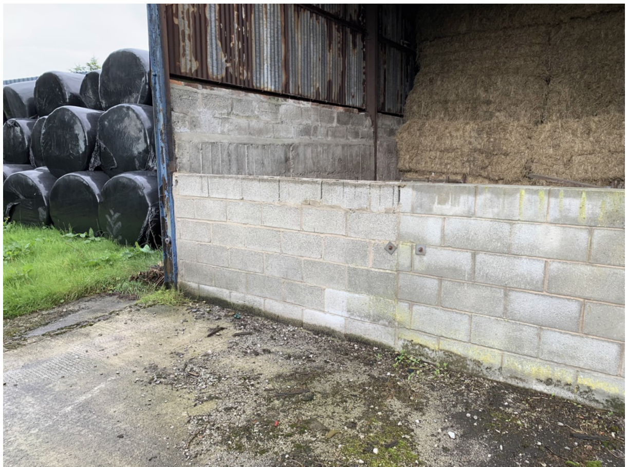
Photo 2 – South Gable - blockwork
