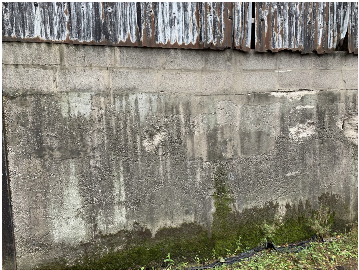
Photo 5 – East Elevation – concrete & block wall
