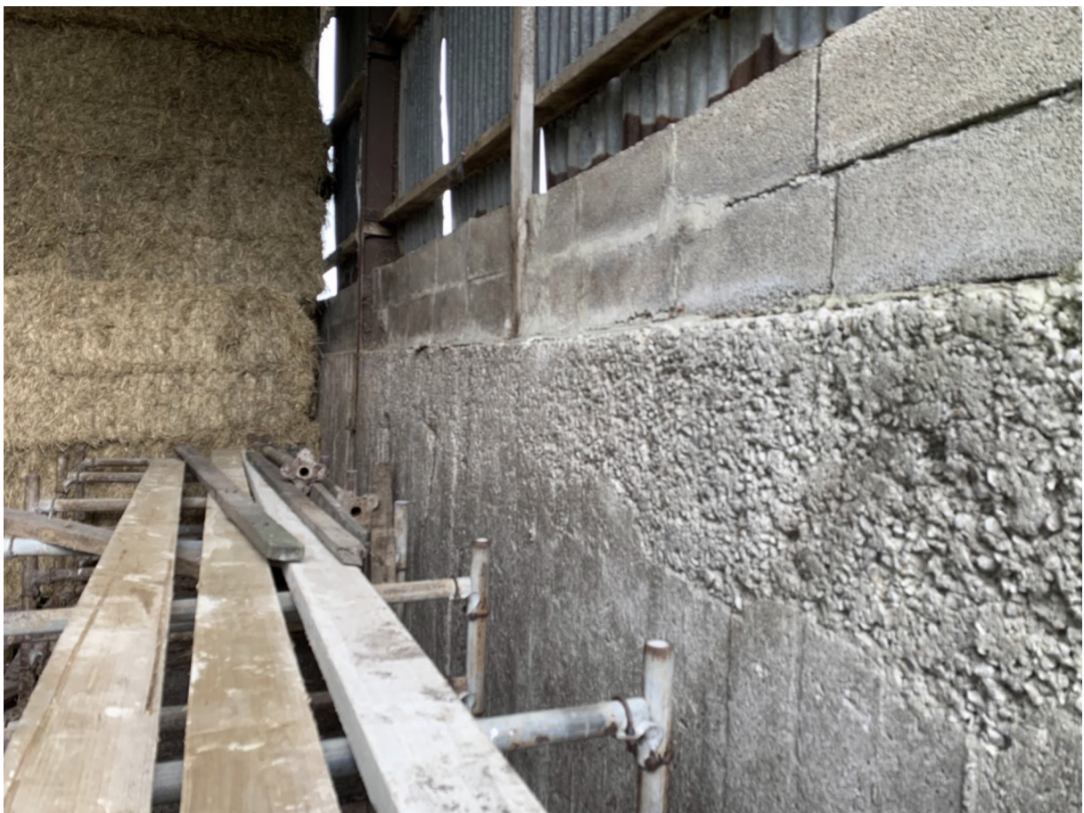
Photo 14 - Internal showing concrete wall
