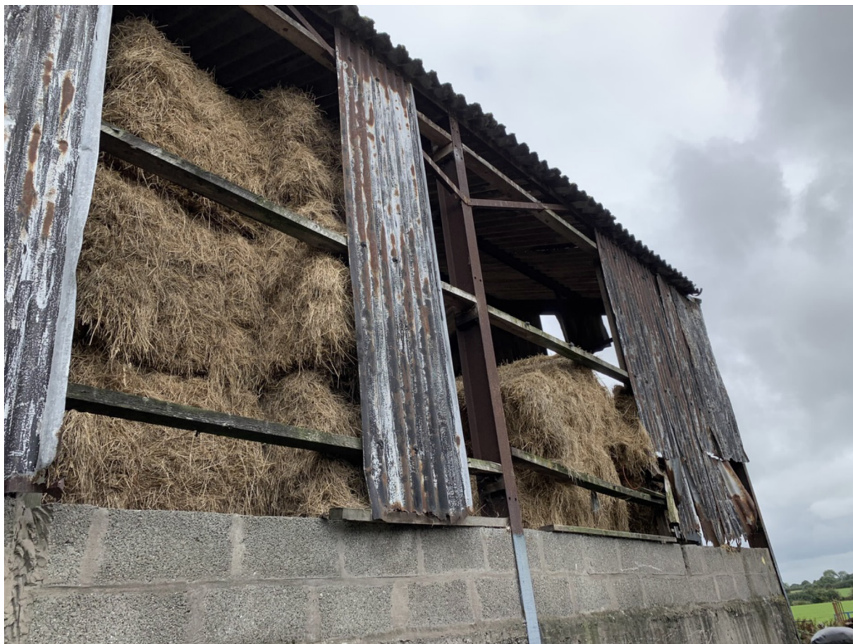
Photo 7 – East Elevation Cladding
