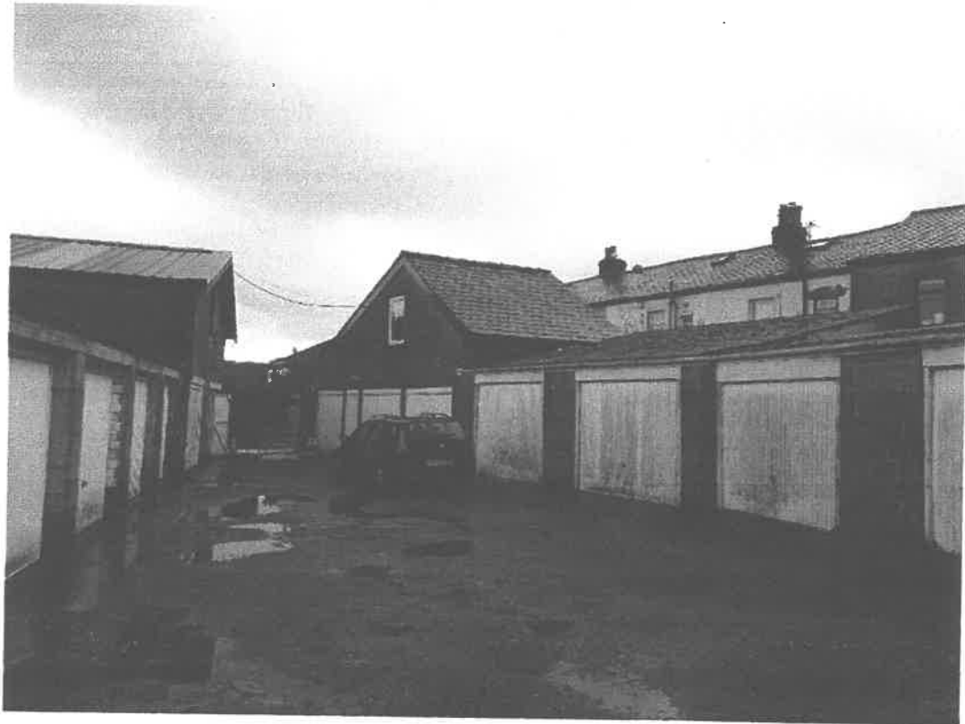
Figure 1: Photograph of the existing garages off Davis Street, facing east
