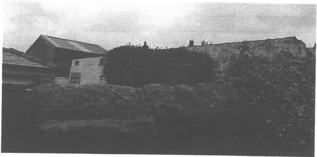
Figure 3: Photograph of the rear of a single storey garage, showing the existing boundary wall
