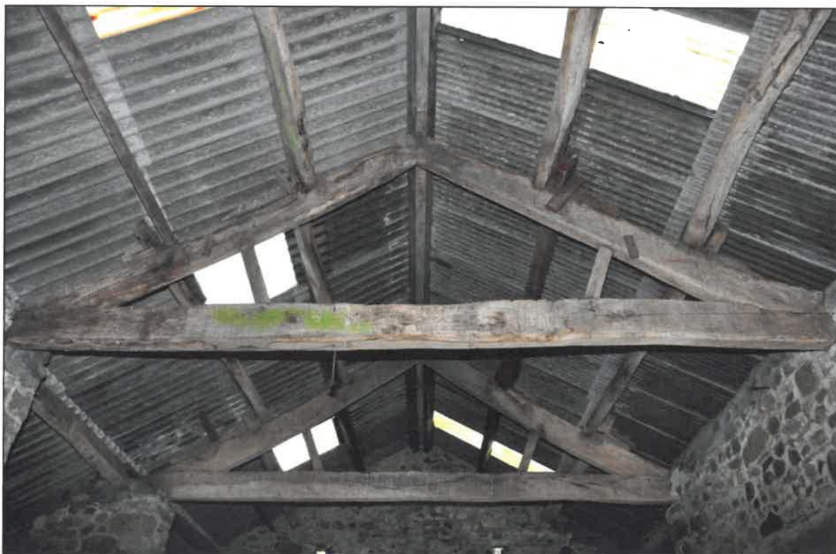
Photo 8: Barn roof structure
