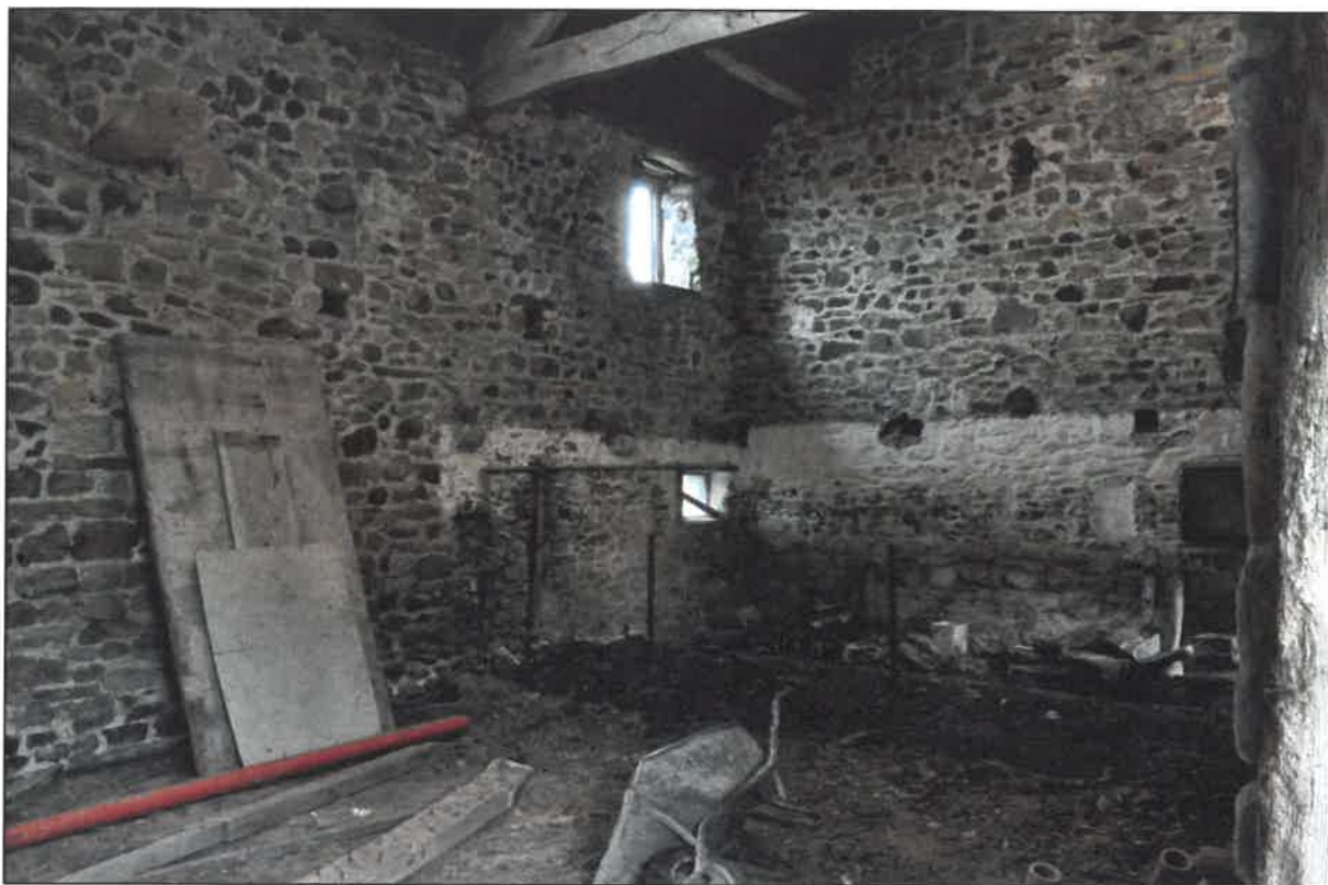
Photo 7: Interior, looking north-east towards site of smaller shippon
