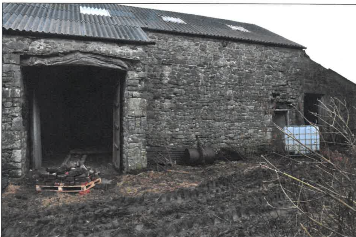
Photo 2: South elevation. Note form of main doorway
