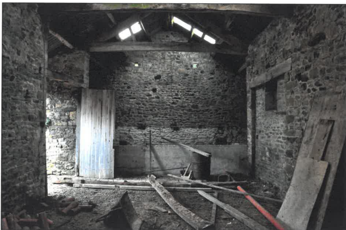
Photo 6: Interior, looking west towards main shippon. Note blocked doorway at right
