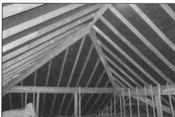
View of closed timber soffit (lhs) and internal view of roof void with timber supports and bitumastic liner (rhs)
