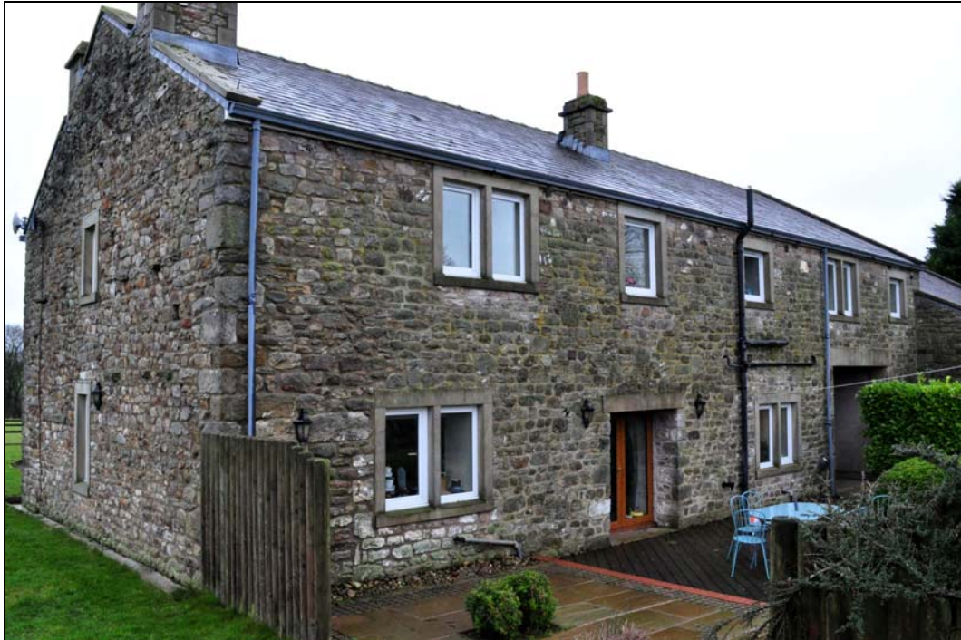
Photo 5: Rear elevation. Some historic fabric evident, but all visible openings are modern.
