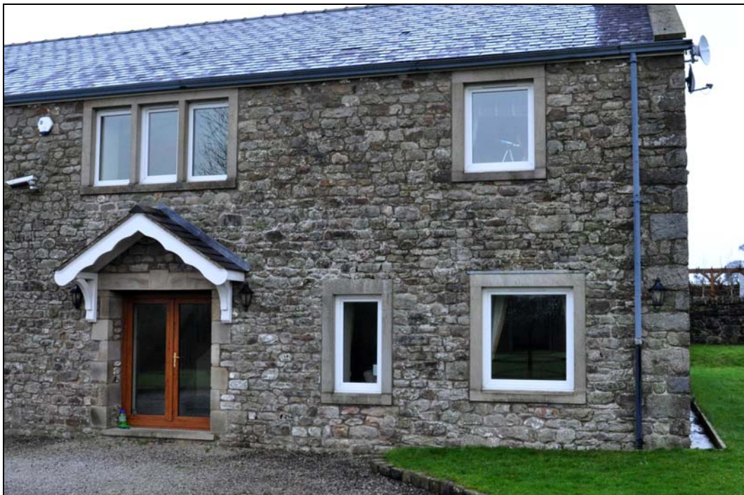
Photo 4: Front elevation with windows (lower right) proposed for replacement by single, floor to ceiling window.
