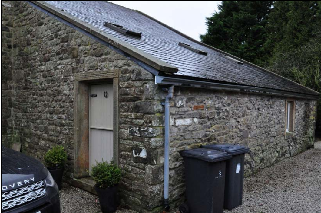
Photo 7: Rear outshot. New window proposed at left. It is recommended that the existing door surround be re-used, for the new opening proposed further left.
