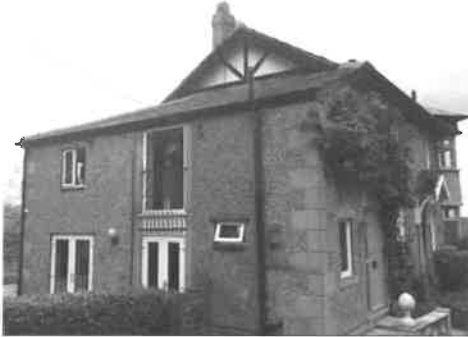
North east gable extension
