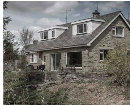
FIG 09 - South West Elevation and Rear Patio
