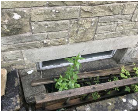
FIG 07 - North West Elevation displaying Basement Window
