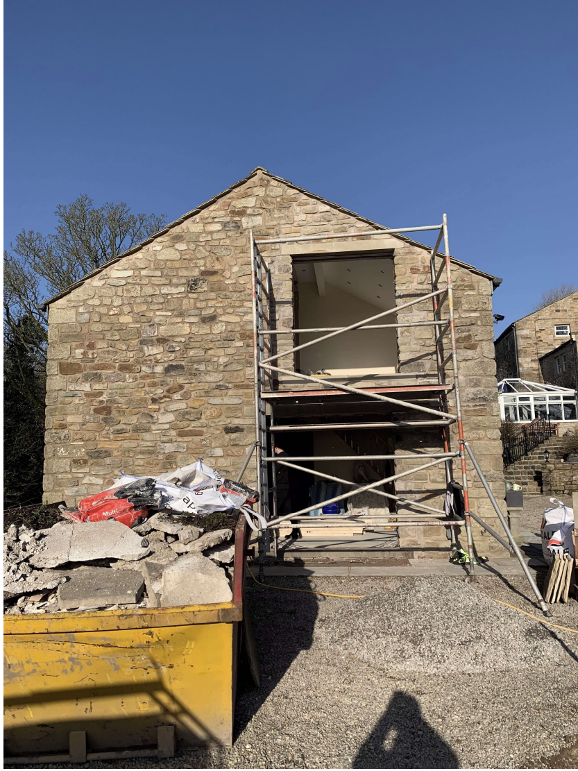
View of the south gable.
