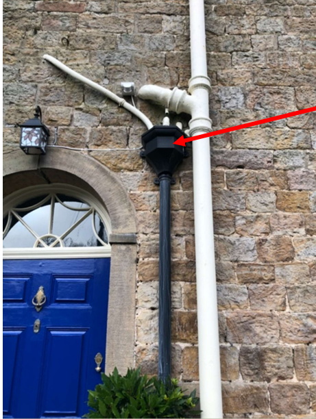
Photo 2- Poorly arranged and inappropriate plastic pipe-work adjacent to the front door
