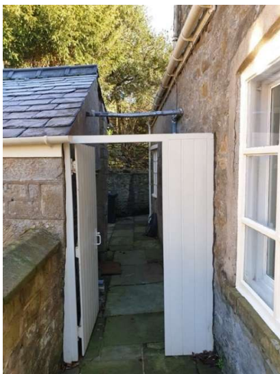
Photo 7 – Existing gate linking wash-house to kitchen
